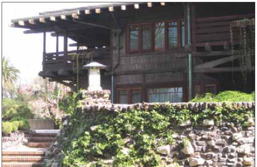
Figure 22 Japanese details at Gamble House include the long rafter tails and the landscaping. These elements are also identified as Arts & Crafts and Craftsman details.
