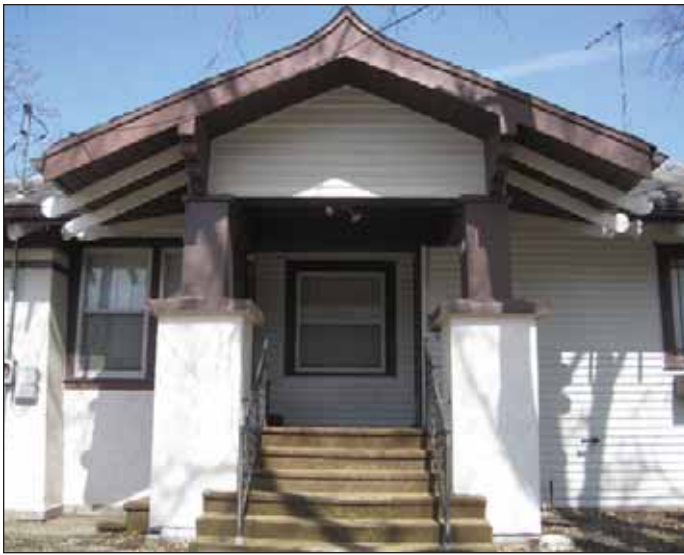
Figure 12 The Arlington Street entrance porch contains both the peaked roof and the circular "ball" rafter end that Burr used to suggest a Japanese influence.
