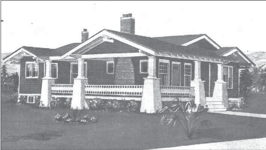
Figure 23 Note the battered columns, open porches, and exposed rafters in this pattern book bungalow. Aladdin "Built in a Day" House catalog, 1917, 29.
