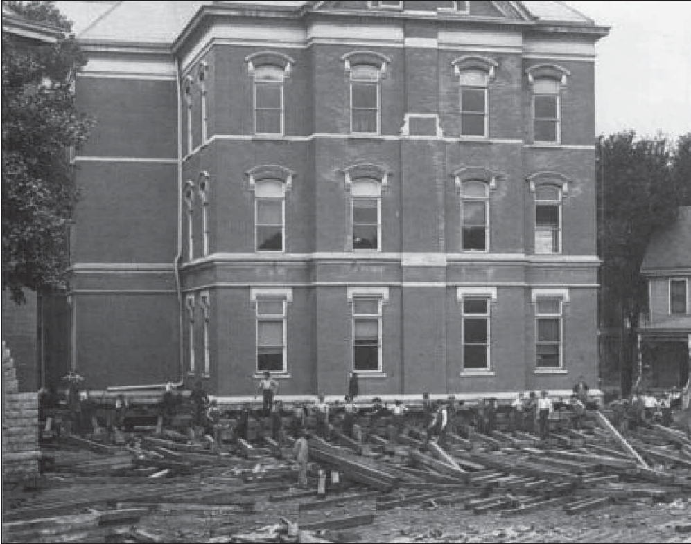
Figure 3 The three-story Science Hall (now Calvin Hall), built in 1885, was moved across the street in 1905 using horsepower and rolling logs. From John C. Gerber, A Pictorial History of the University of Iowa (1988).
