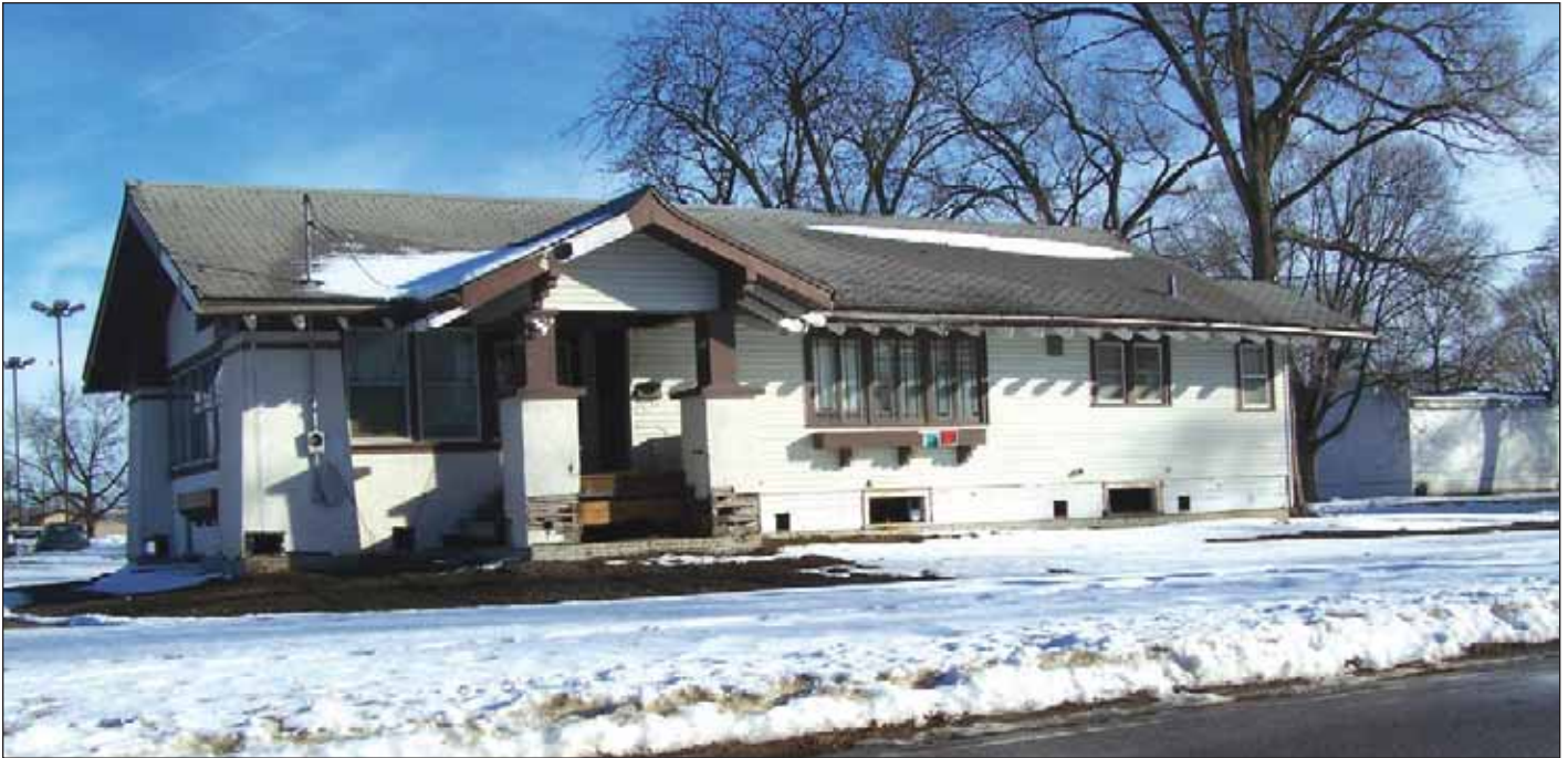
Figure 44 The front porch is on the left and now overlooks empty lots. The back door is on the right and overlooks a city street. The house has not been renovated on the new site. Photo supplied by Chris Western, City of Waterloo, December 2013.
