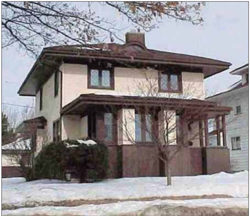
Figure 35 This basic Foursquare has been rendered a stylish Prairie School residence by the addition of its very wide eaves on the shallow roof of both the house and the porch. Black Hawk County Assessor photograph.
