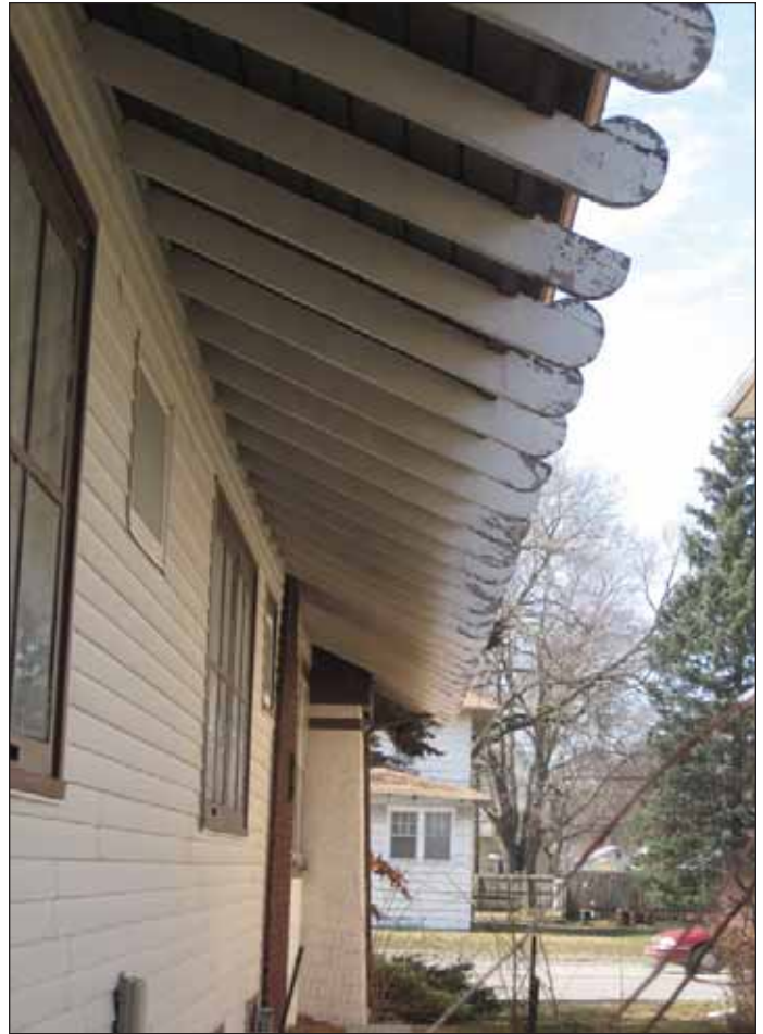
Figure 13 Exposed rafter ends were meticulously fitted with rounded pieces to suggest a flared eave. Here, the north side of the house has lost some of these pieces to the elements over time.
