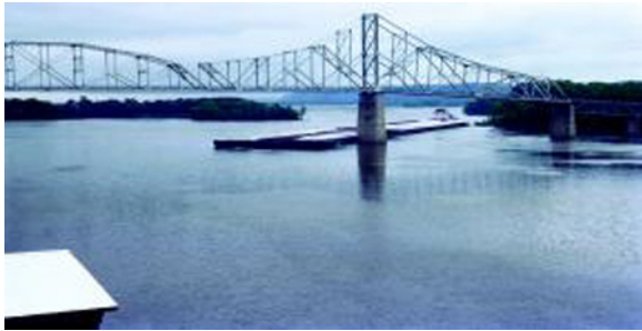
The Actual hit of the pier resulting in the break away string of barges shown in the next two snapshots.
