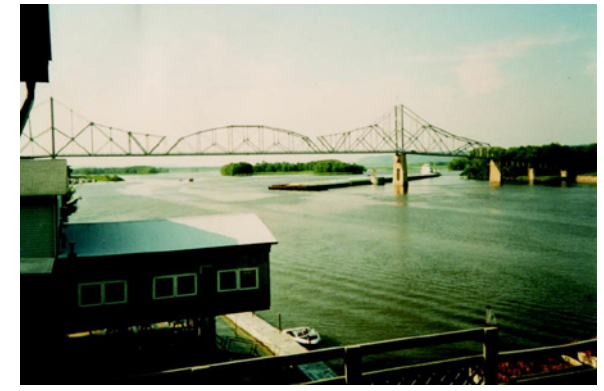
1994 - A tow resting against dolphin (dolphin built in 1992).
