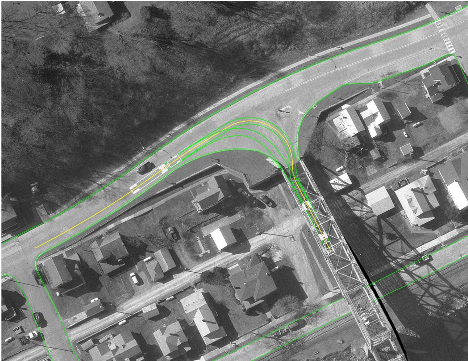
Northbound to eastbound truck turning movement at the intersection of IA 9/IA 26 and the Black Hawk Bridge
