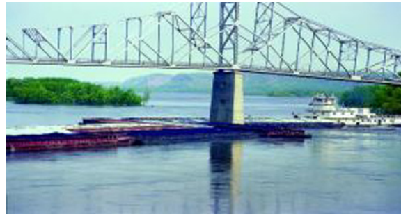
The barges coming apart after cables snapped.
