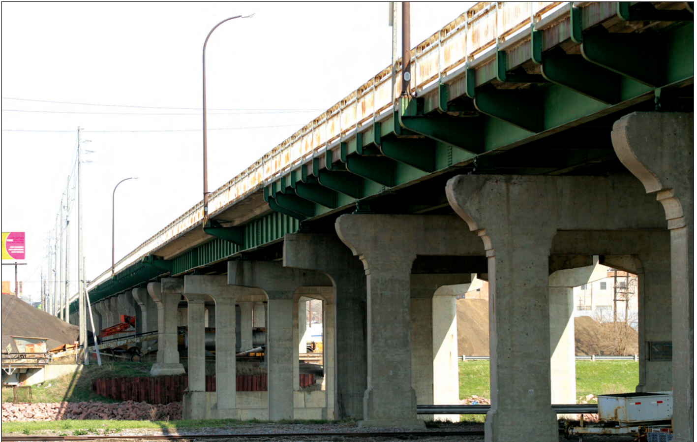
North side of the Grand Avenue Viaduct, looking southeast. The line of original curved piers is interrupted by the "T" piers and three spans built in 1963 over the relocated Floyd River channel.
