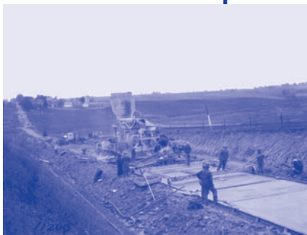
Paving the Lincoln Highway East of Colo c. 1928. Note use of larger gasoline driven concrete mixer by this time. Photo Courtesy: Iowa Department of Transportation, Ames
