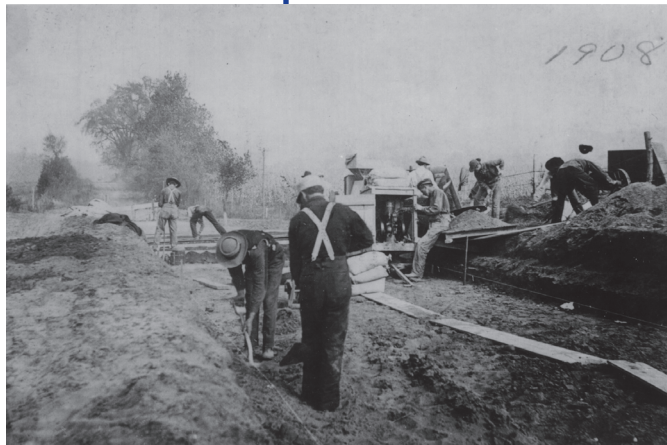
1908 Photo of concrete paving near Eddyville, Iowa. Note use of hand mixer. Photo Courtesy: State Historical Society of Iowa, Des Moines.
