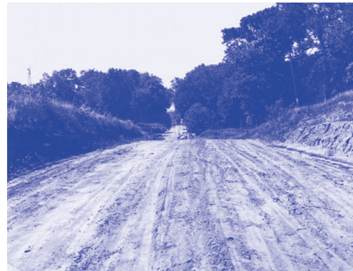
1918 Photo of grading for Linn County Seedling Mile. View to northwest from mid-section of mile. Photo Courtesy: Iowa Department of Transportation, Ames
