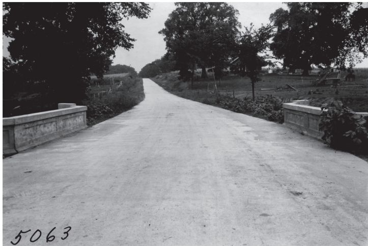
1921 Photo of East end of Linn County Seedling Mile view to northwest. Note Harry Stoneking's bungalow on right. Photo Courtesy: Iowa Department of Transportation, Ames
