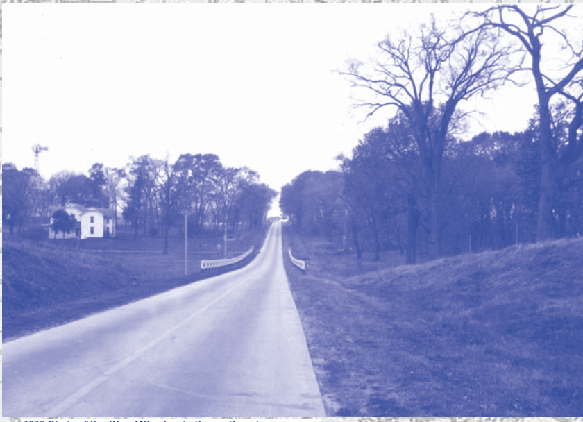
1928 Photo of Seedling Mile view to the northwest. Photo Courtesy: Iowa Department of Transportation, Ames
