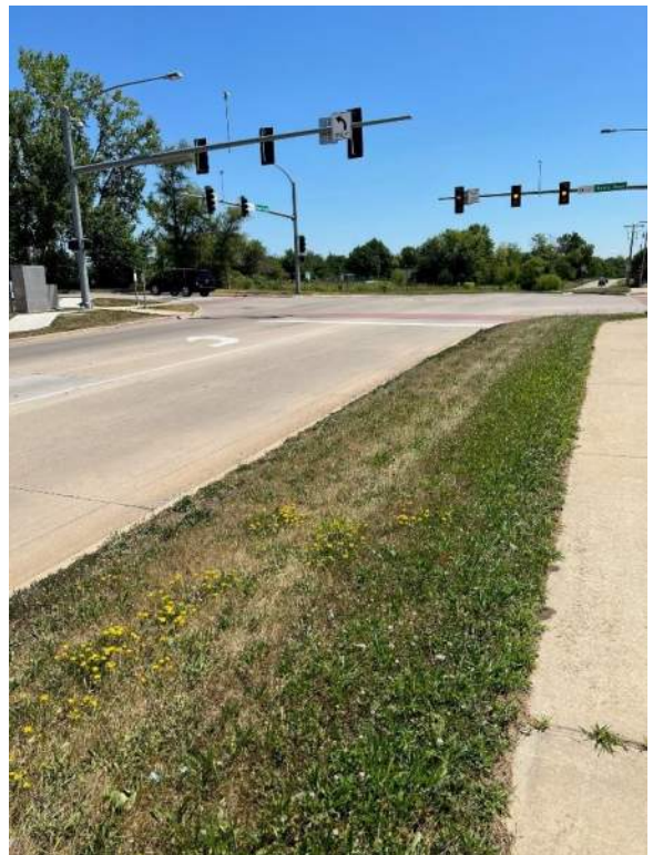
Boyson Road 3-lane section west of Robins Rd
