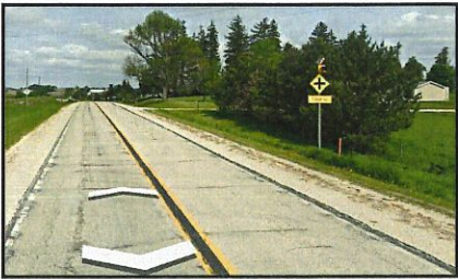
IA 56 Westbound has an intersection ahead flashing beacon
