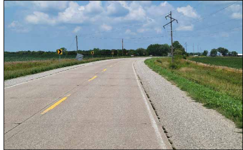
Photo 5: Typical curve section (note inside edge rutting).
