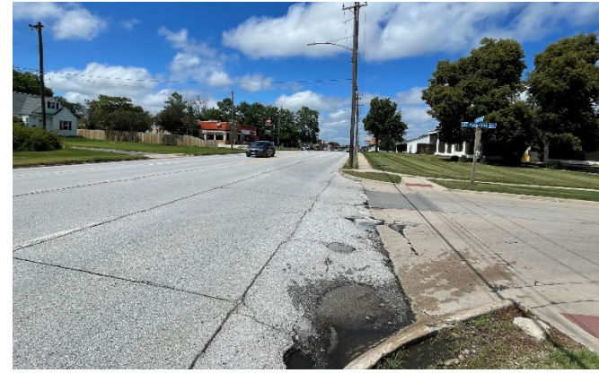
S Ankeny Boulevard viewing North at SE Peterson Drive
