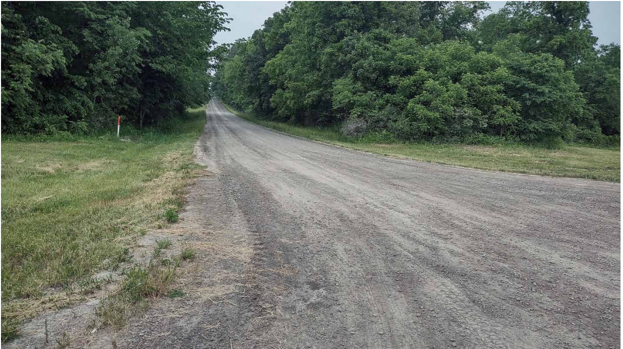
210 TH STREET WEST FROM HWY 1
