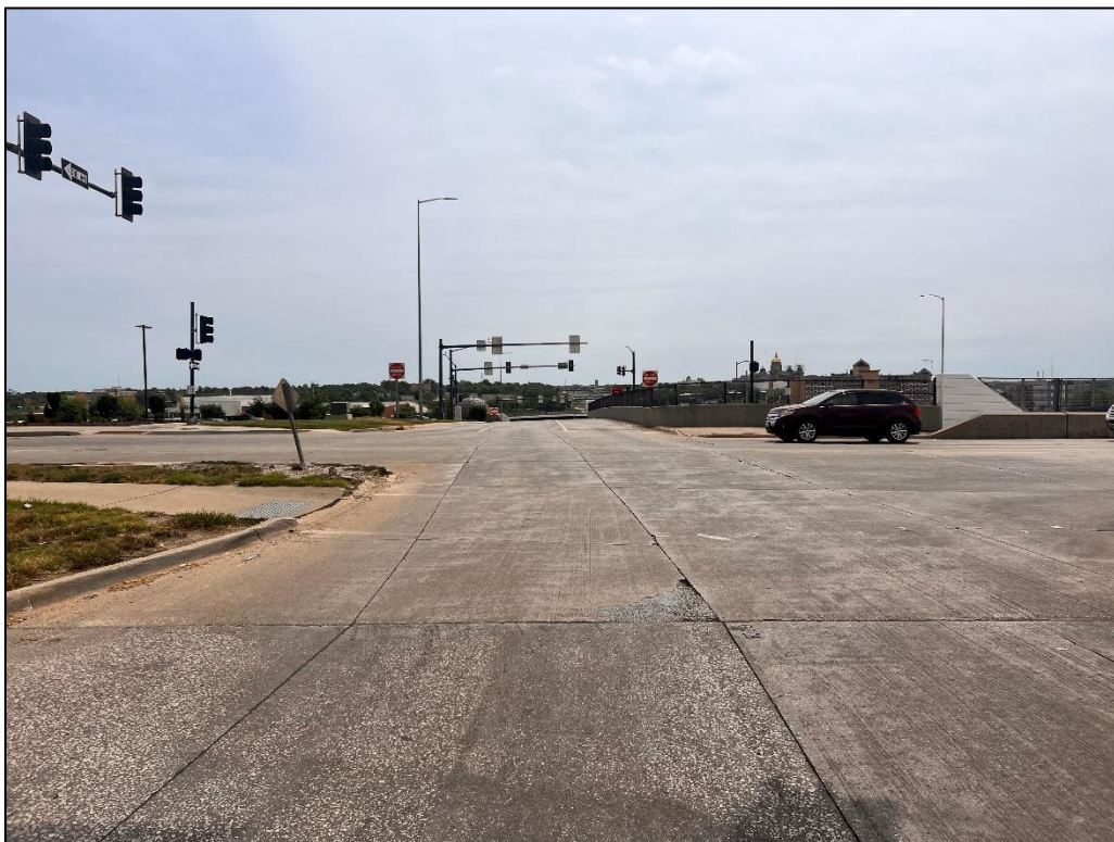
Day Street – Looking East
