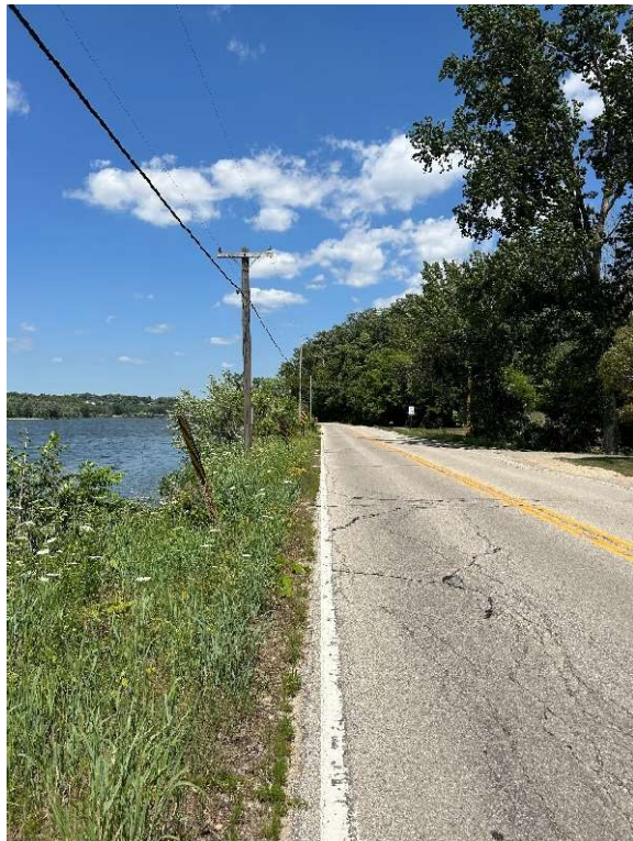
Figure 2: Typical roadway segment with no guardrail
