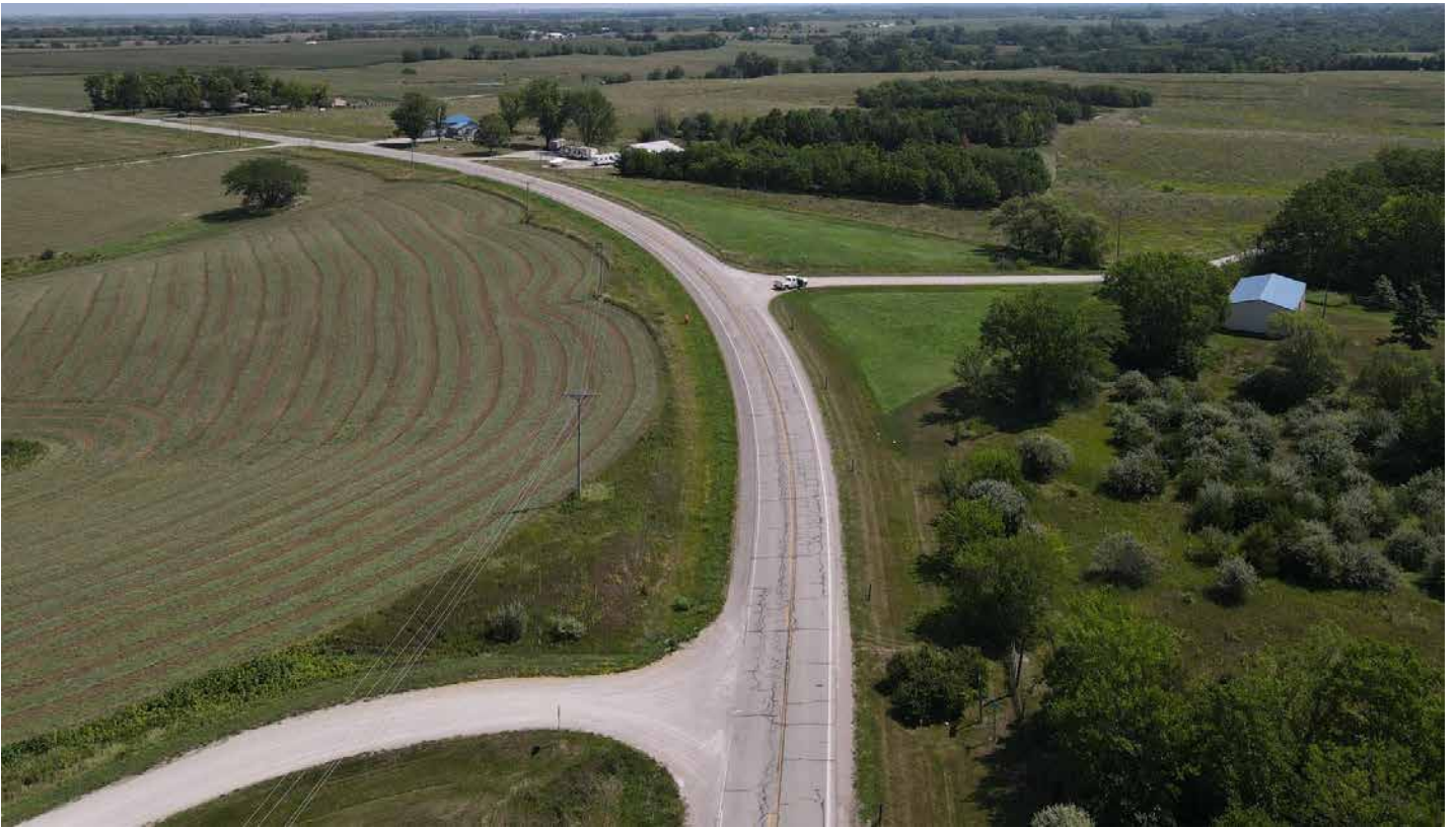
Site A looking north
