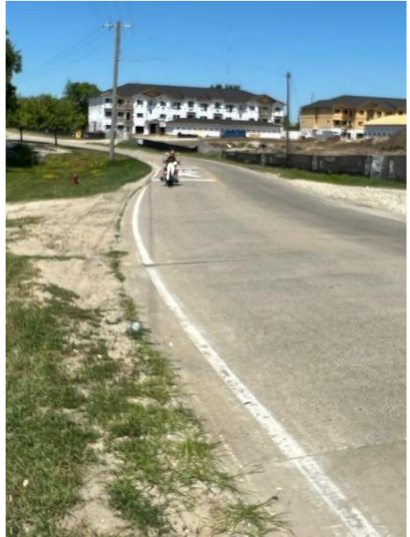
Boyson Road between Hawkeye Drive and railroad crossing
