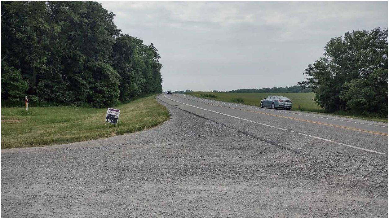
HIGHWAY 1 SOUTH FROM NORTHERN DILLONS FURROW INTERSECTION
