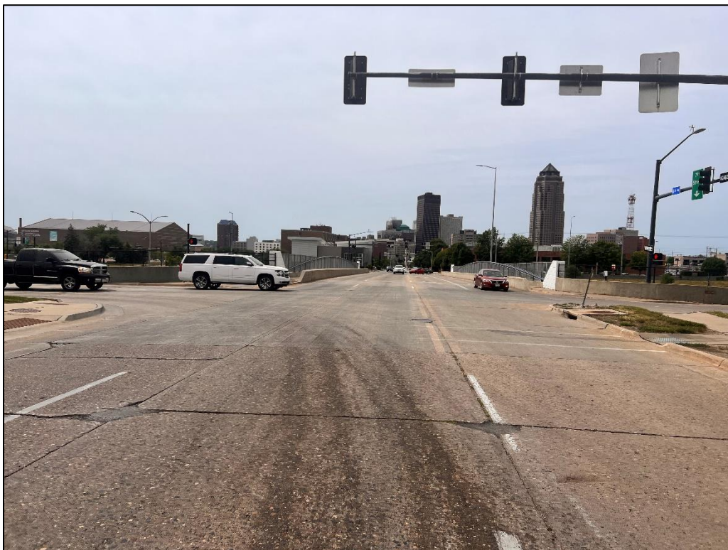
6 th Avenue – Looking South
