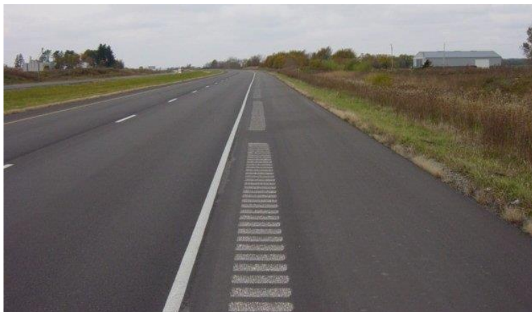
Figure 3: Gapped shoulder rumble strip pattern.
