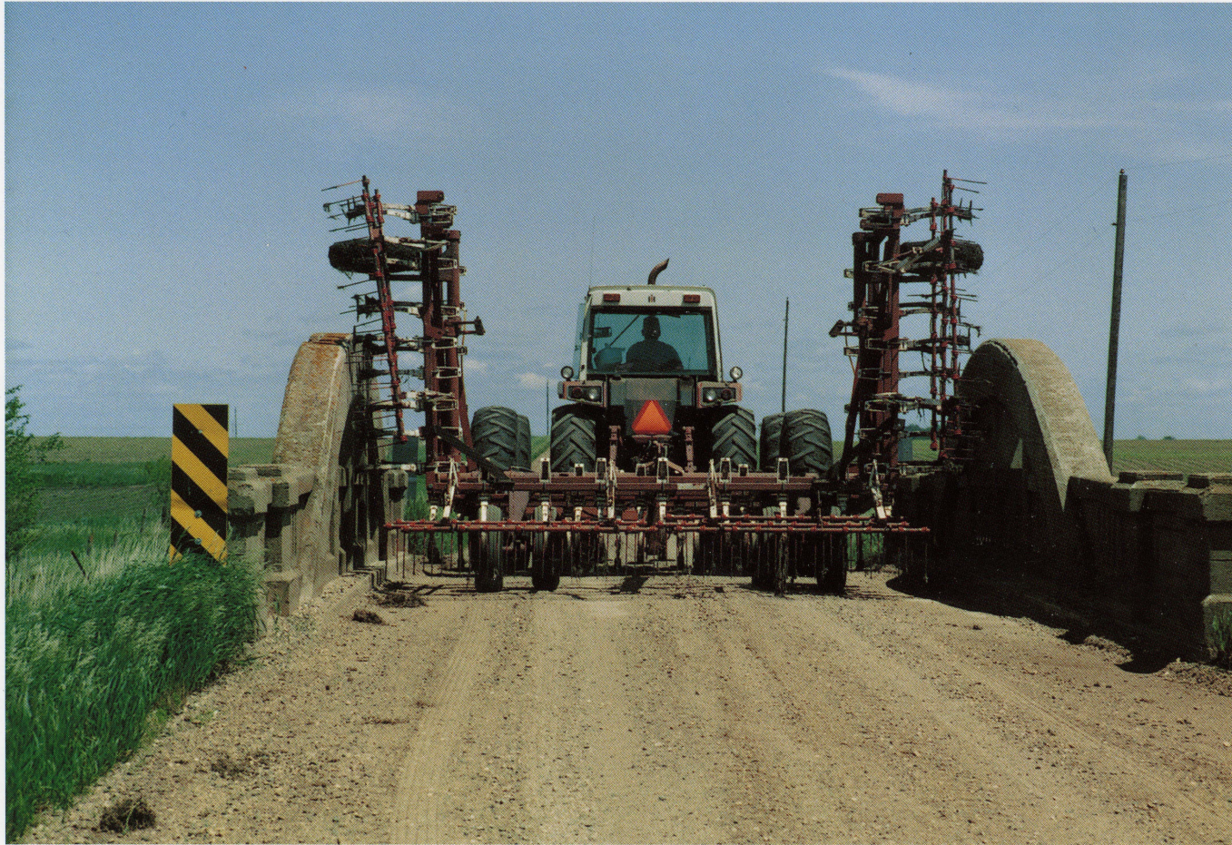
A tractor just clears a Boone County arch – Beaver Creek Bridge (North), Boone County
