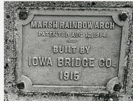
Builder's plate on Rockwell City Bridge. The patent date is apparently incorrect.
