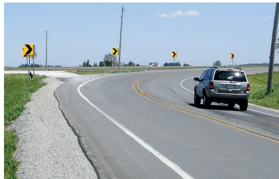
Installation of larger chevrons and other low cost remedies help reduce crashes on state and local roads identified in a recent TSIP project.
