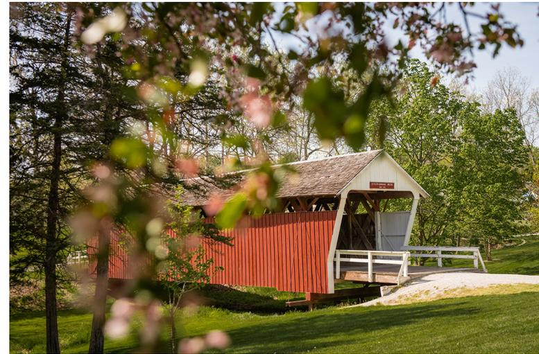
“One of the first covered bridges Eli Cox built was the Donahue bridge over North River near the eastern line of the county. The cover protects the timbers and prevented rain from getting into the joints and around nails and bolts. There are still a number of these bridges in the county and people drive from afar to see them.” *Winterset Madissonian*, July 13, 1949
