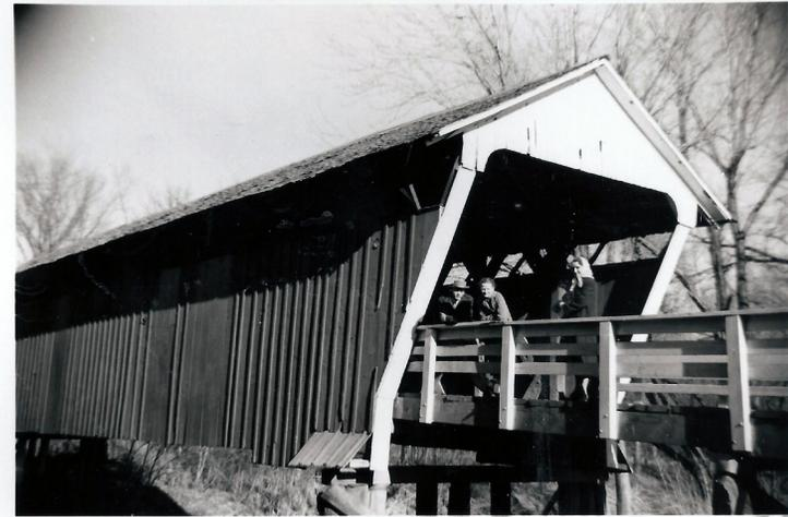
Mueller continues, “One of the first covered bridges Eli Cox built was the Donahue bridge, over North River, near the eastern line of the county. It stands here today a testimony to his honest workmanship. The cover protected the timbers and prevented rain from getting into the joints and around nails and bolts. When these old bridges are taken down the timbers are invariably found to be in a good state of preservation.”
