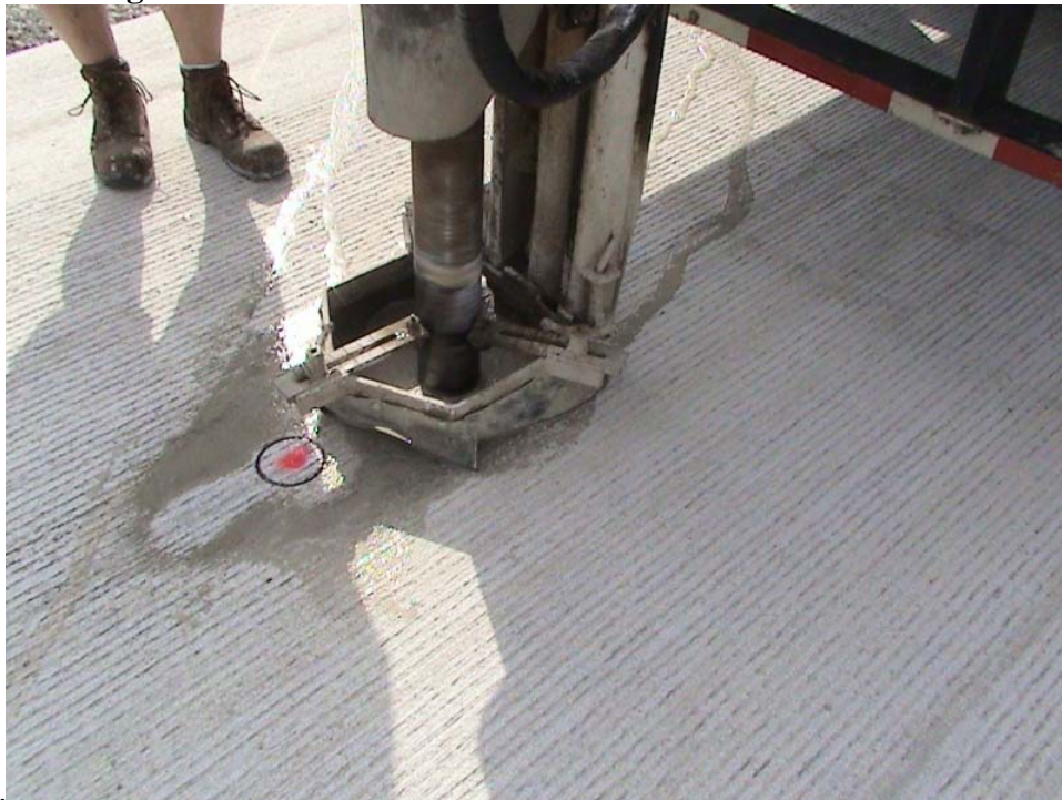
Figure 4 Coring at test locations.
