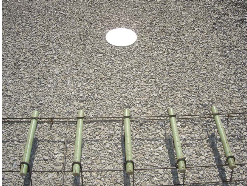
Figure 1 Target placed on granular subbase.
