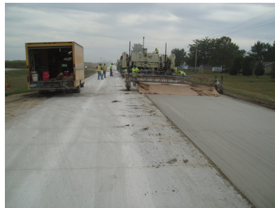
Single-lane stringless paving in Worth County
