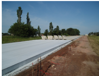
Finished pavement in Osceola County
