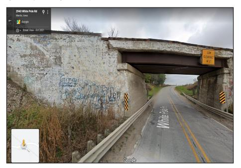
The WPR Board recommends informing the IAIS of its condition and inquiring about possible plans to repair it. The issue of the graffiti is a more complex one as it may require frequent repainting of the concrete on both sides of the structure.
