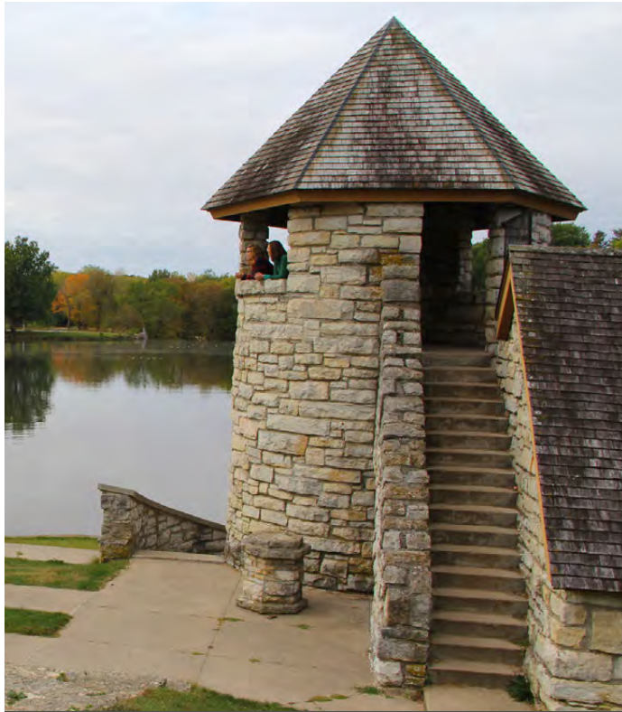
CCC Boathouse Structure
