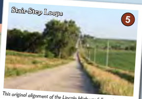
5 Scurt-Step Loops This original alignment of the Lincoln Highway followed surveyed section lines, making right-angled turns at every corner. As cars got faster, curves were engineered into the corners for safety.
