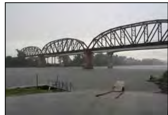
1924 Union Pacific Railroad bridge over the Missouri River
