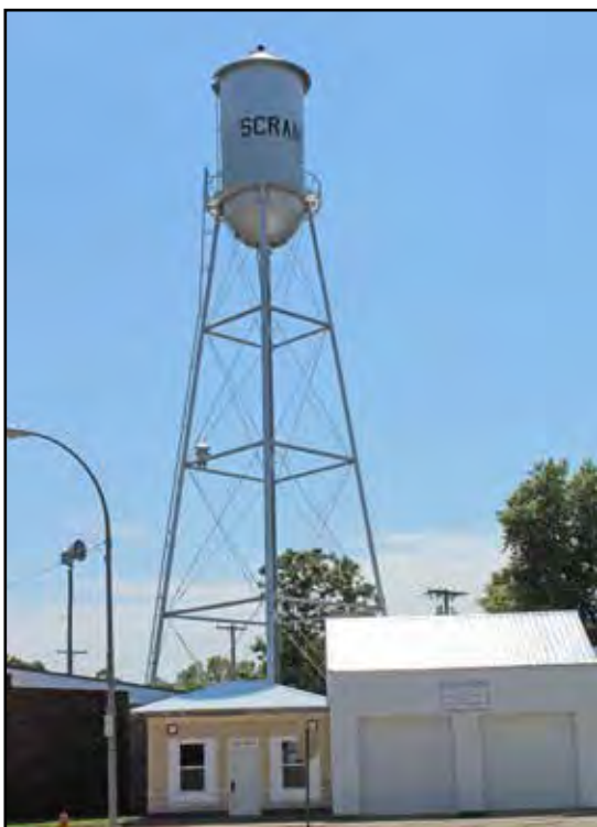
1897 Scranton Water Tower
