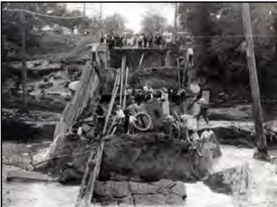
Squaw Creek bridge collapse in Ames, 1918
