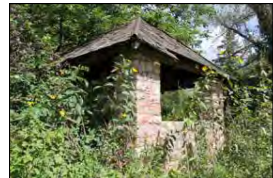
Meskwaki Stone Well House
