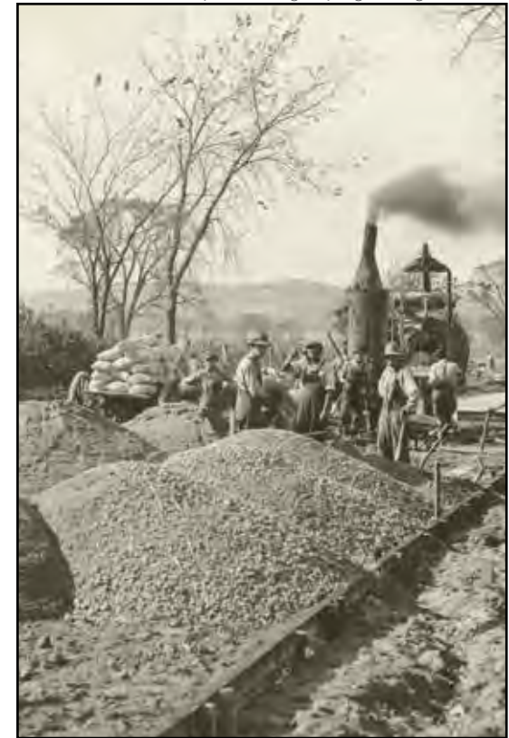
Concrete construction underway on the Lincoln Highway in central Iowa, 1915
