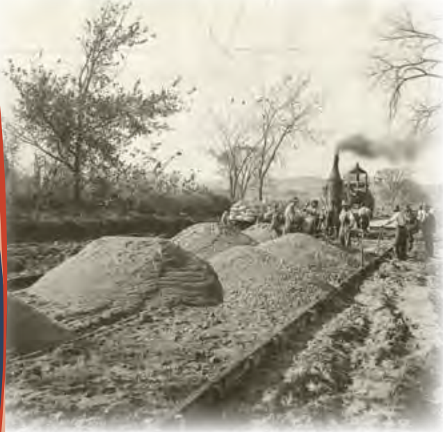
Concrete construction underway in central Iowa, 1915
