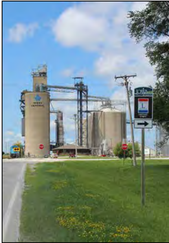
Scene along the Lincoln Highway Heritage Byway, Jordan, Boone County
