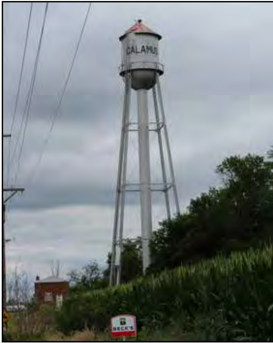
Calamus water tower
