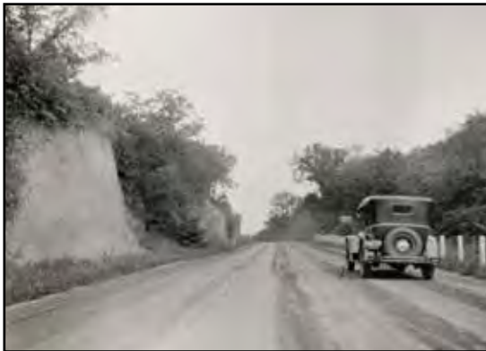
The Loess Hills created challenges for the early Lincoln Highway, requiring deep hill cuts, like this one at Honey Creek Hill north of Crescent.
