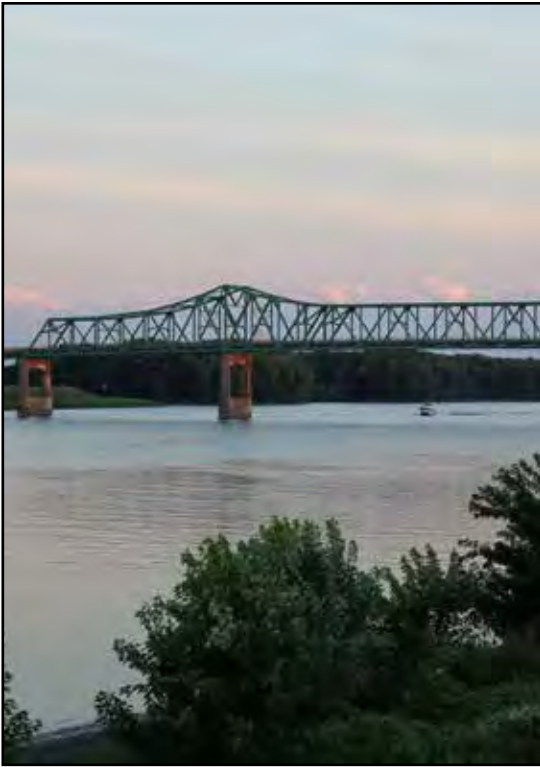
View of the Highway 136 bridge on the Lincoln Highway, which crosses the Mississippi River between Illinois and Iowa
