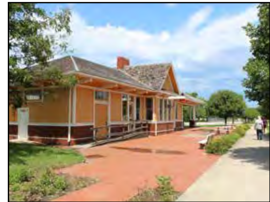
Restored Milwaukie Railroad Depot in Jefferson
