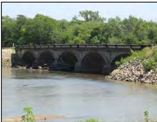
1913 Eureka Arch Bridge over the Raccoon River
