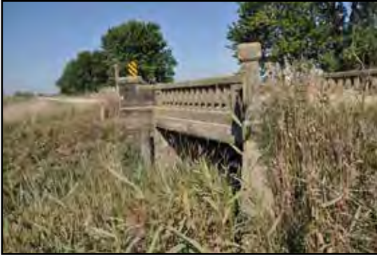
1915 "L" Bridge over Beaver Creek
