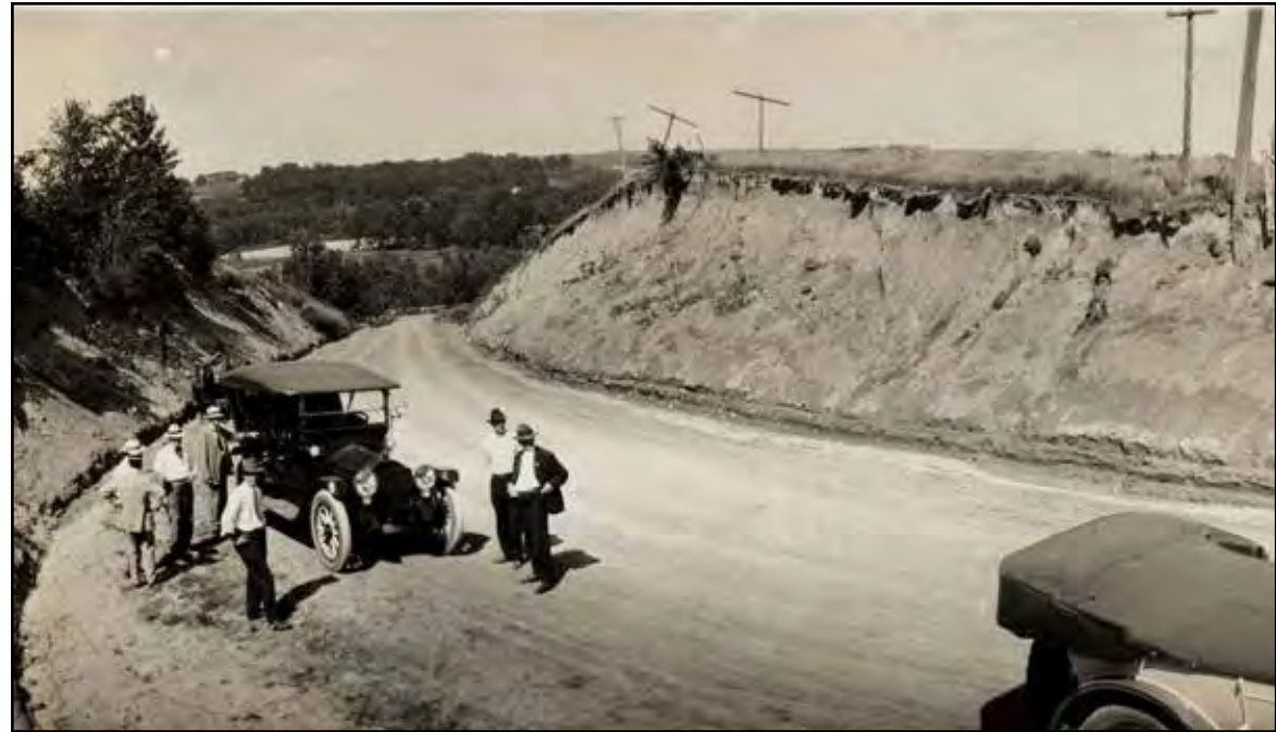
Heavy cut work and grading reduced the slope of Danger Hill west of Jefferson, 1918
