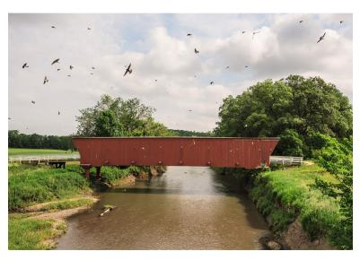
The Hogback Bridge was also built by Harvey P. Jones and George K. Foster using the Town lattice truss with queenpost overlay. It was the last covered bridge built in Madison County. The Hogback spans 98 feet over the North River, four miles northwest of Winterset. While most of the covered bridges were named for nearby landowners, the Hogback was named for the Hogback Ridge at the west end of the valley (its convex curve resembling the curve of a hog's back).
