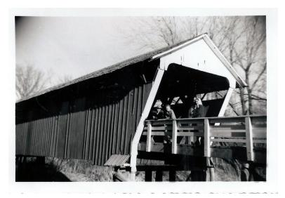
Mueller continues, "One of the first covered bridges Eli Cox built was the Donahue bridge, over North River, near the eastern line of the county. It stands here today a testimony to his honest workmanship. The cover protected the timbers and prevented rain from getting into the joints and around nails and bolts. When these old bridges are taken down the timbers are invariably found to be in a good state of preservation."
