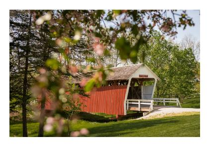
"One of the first covered bridges Eli Cox built was the Donahue bridge over North River near the eastern line of the county. The cover protects the timbers and prevented rain from getting into the joints and around nails and bolts. There are still a number of these bridges in the county and people drive from afar to see them." Winterset Madisonian, July 13, 1949
