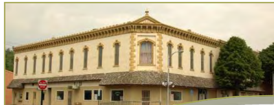
Before & After Façade Improvements
