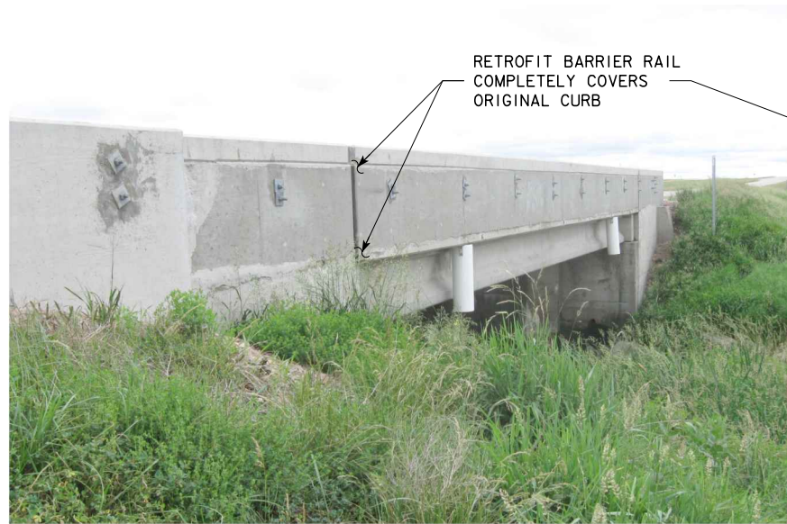
CURB INTEGRATED INTO RAIL
