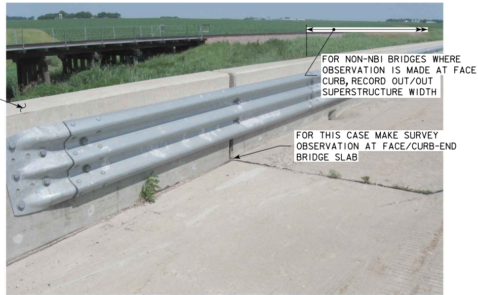
CURB INTEGRATED INTO RAIL
