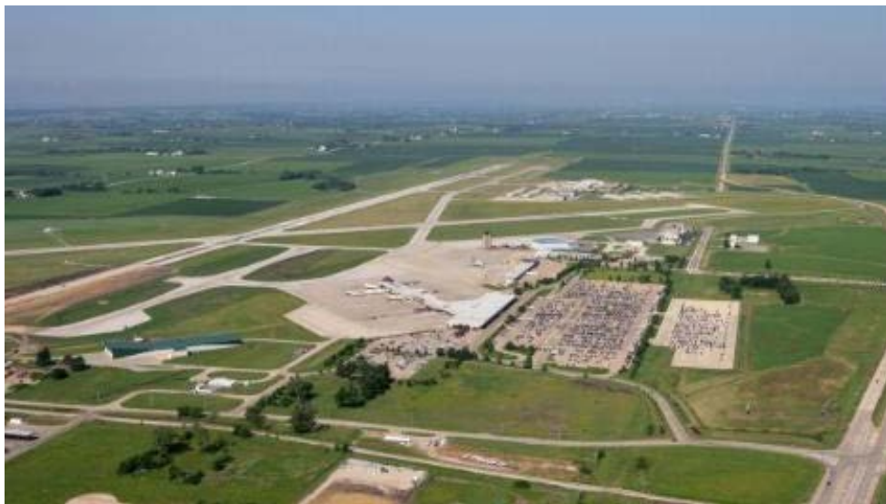
The Eastern Iowa Airport near Cedar Rapids, Iowa, aerial photo looking west with runway construction work on left side and Wright Brothers Boulevard lower right side, 6/23/2006.
