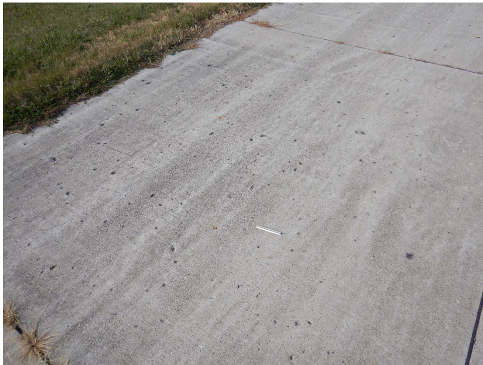
T12AM-01. Popouts (Sample Unit No. 04).
