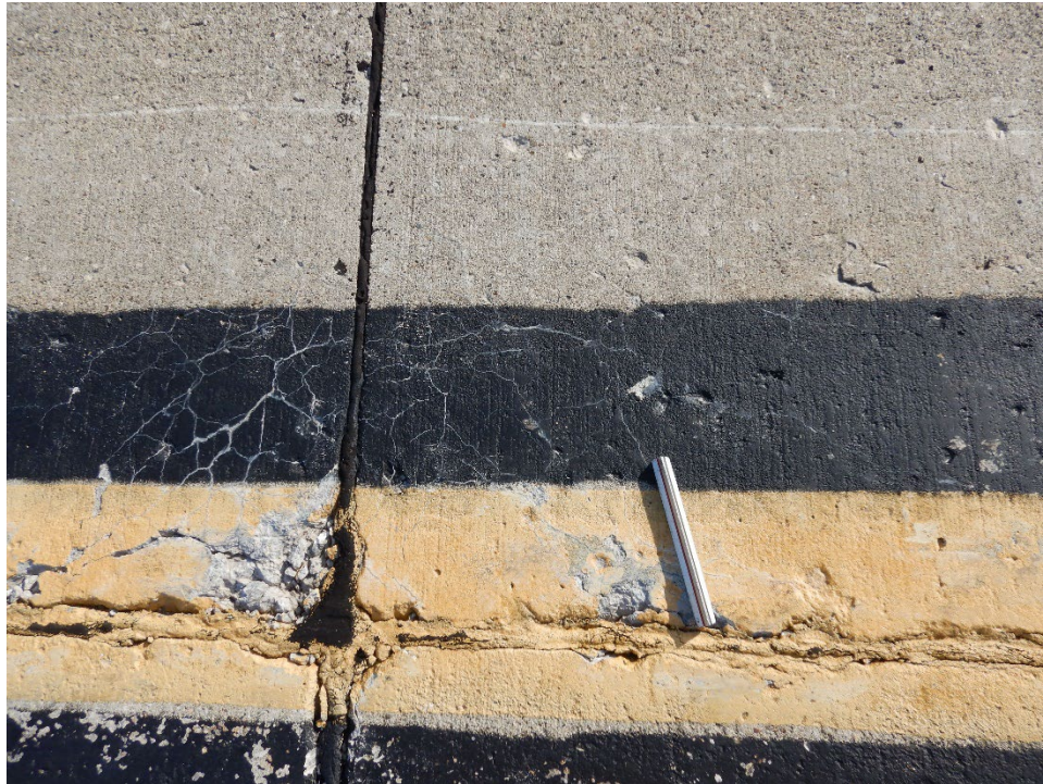
T10AM-01. ASR (Sample Unit No. 24).
