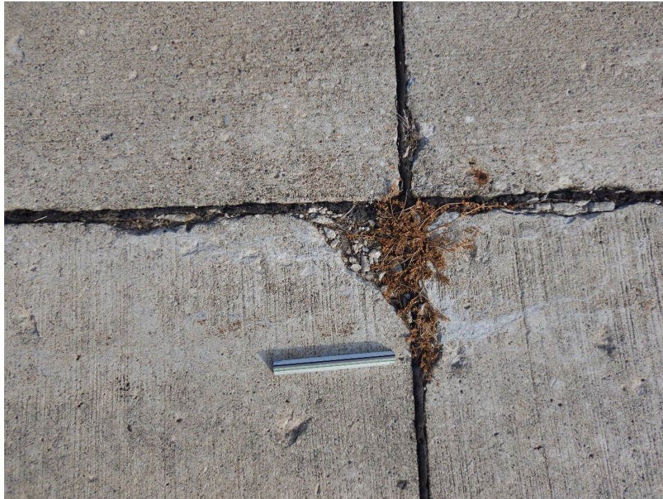
T12AM-01. ASR (Sample Unit No. 04).
