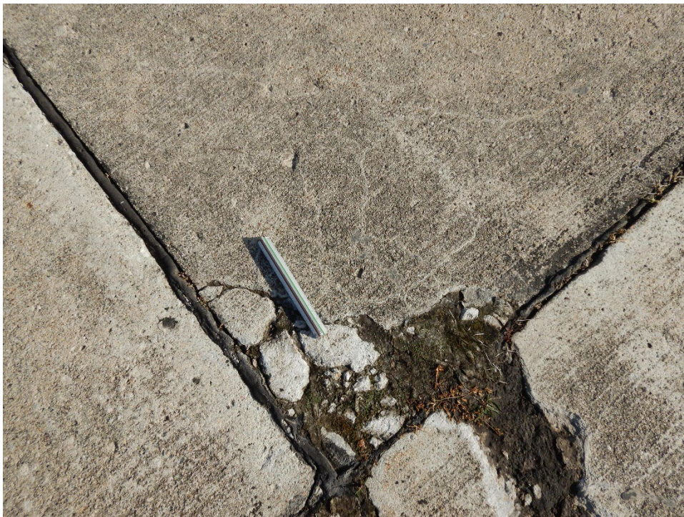
T11AM-01. ASR (Sample Unit No. 06).
