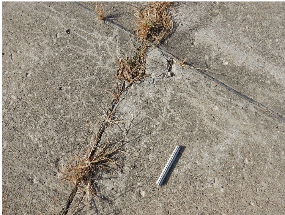
T01AM-01. ASR (Sample Unit No. 05).
