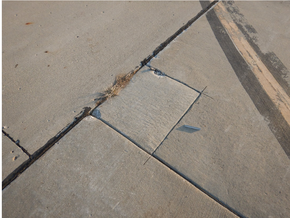
T05AT-01. Small Patching (Sample Unit No. 01).
