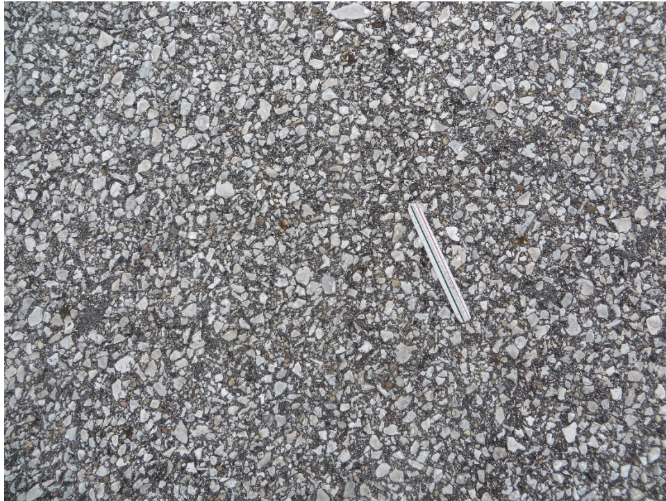
TH01BO-02. Weathering (Sample Unit No. 01).
