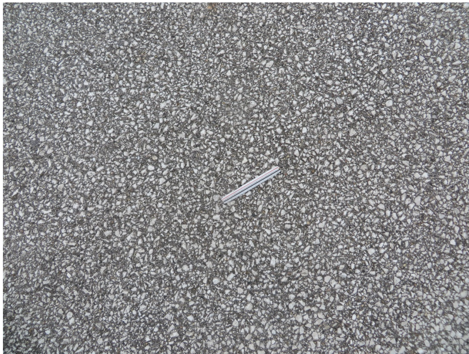
TH01BO-01. Weathering (Sample Unit No. 02).
