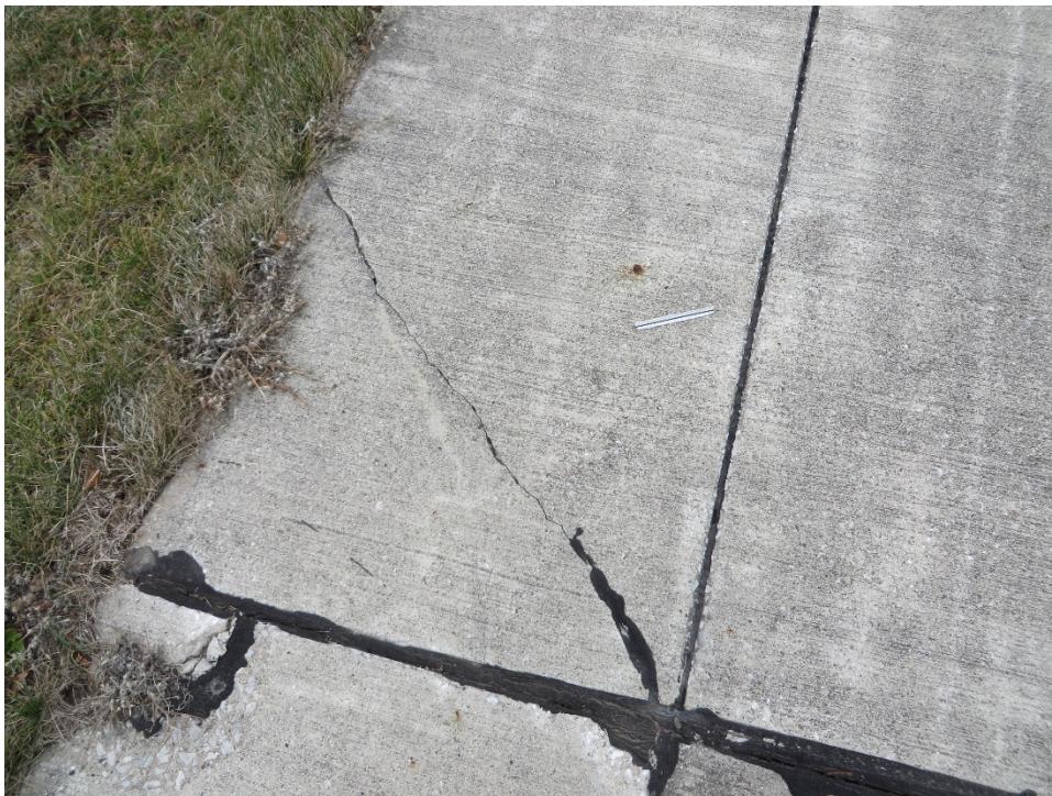
T01BO-06. Corner Break (Sample Unit No. 01).
