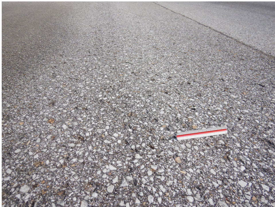
TH01BR-01. Raveling (Sample Unit No. 02).
