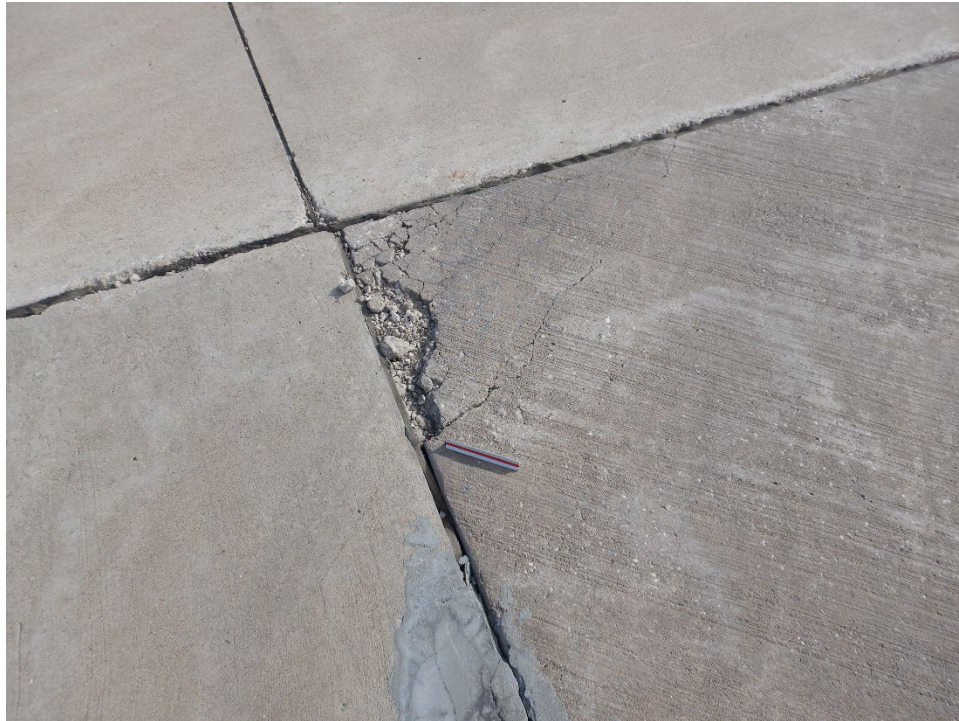
T04BR-01. ASR (Additional Sample Unit No. 11).
