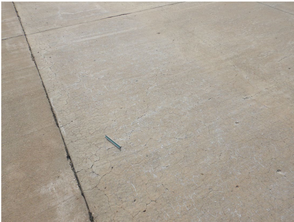
T05BR-02. ASR (Sample Unit No. 03).
