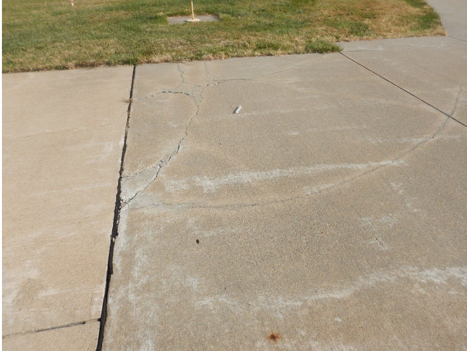
TH01BR-02. Shattered Slab (Additional Sample Unit No. 01).
