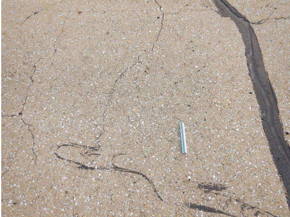
T03BR-04. Raveling (Sample Unit No. 02).
