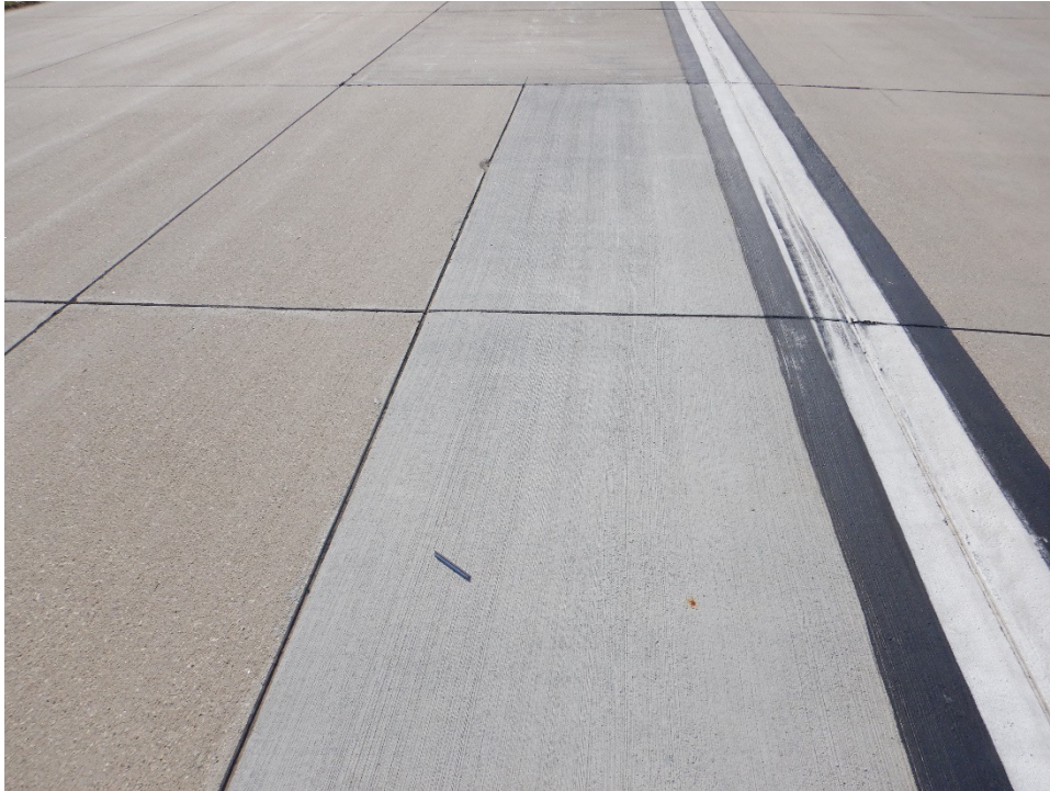
R03CA-01. Large Patching (Sample Unit No. 09).
