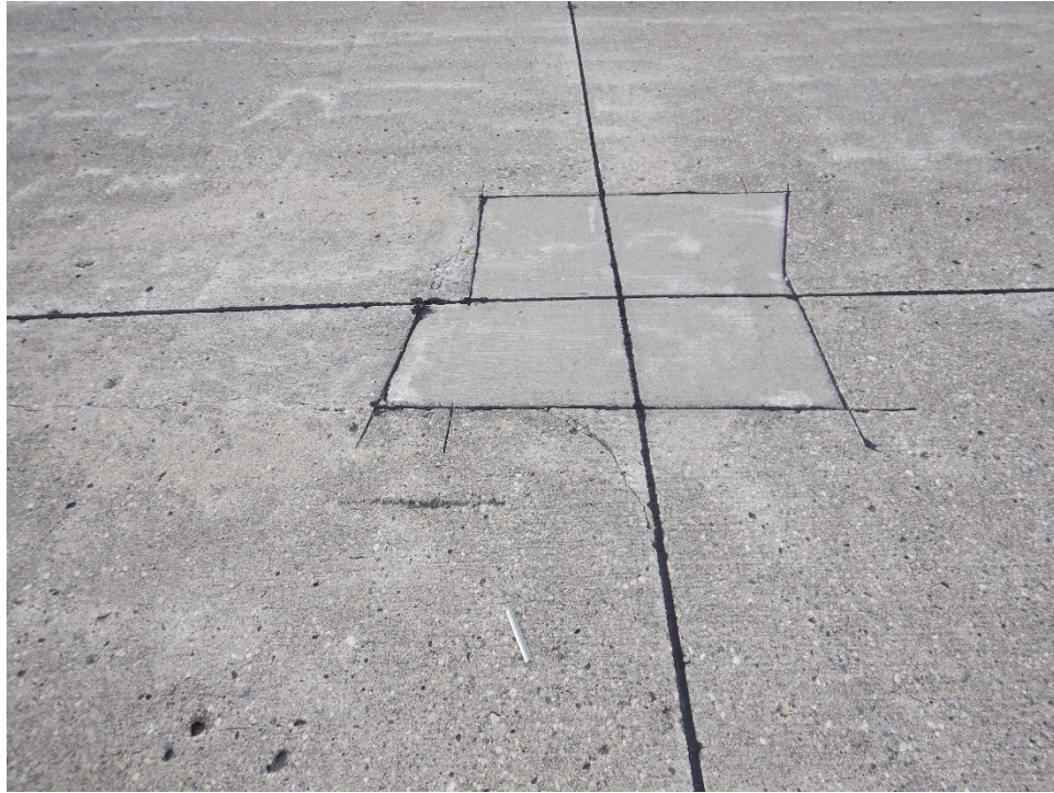
R13CA-02. Small Patching (Sample Unit No. 05).
