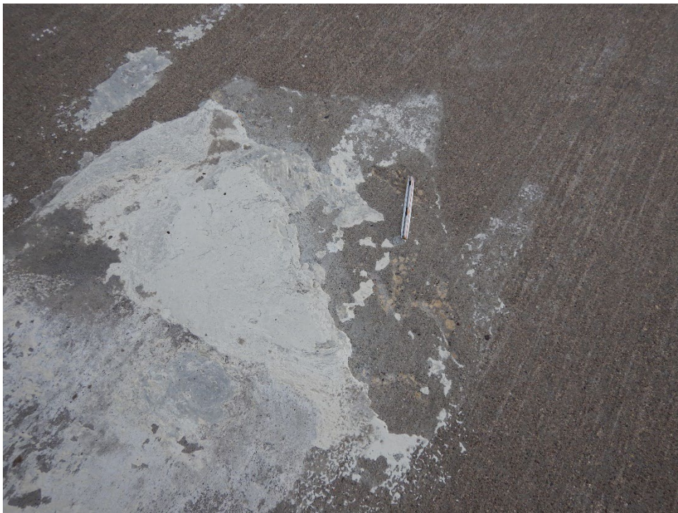
R03CN-01. Scaling (Additional Sample Unit No. 110).
