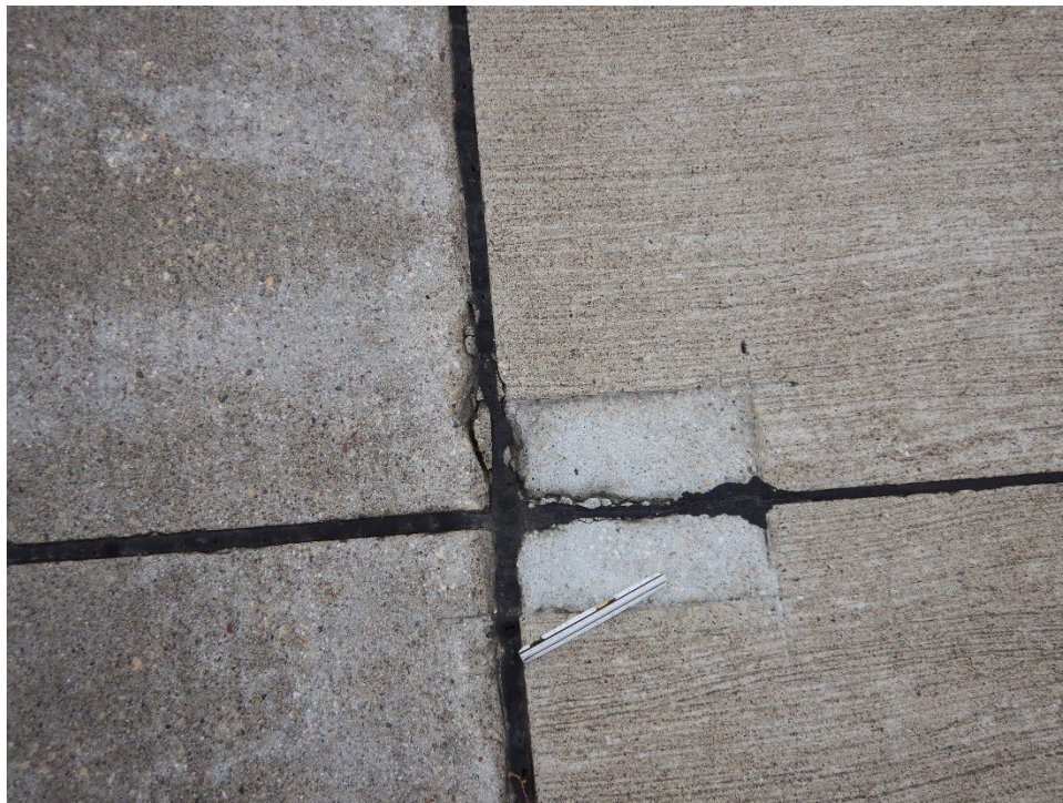
T03CN-02. Small Patching (Sample Unit No. 01).
