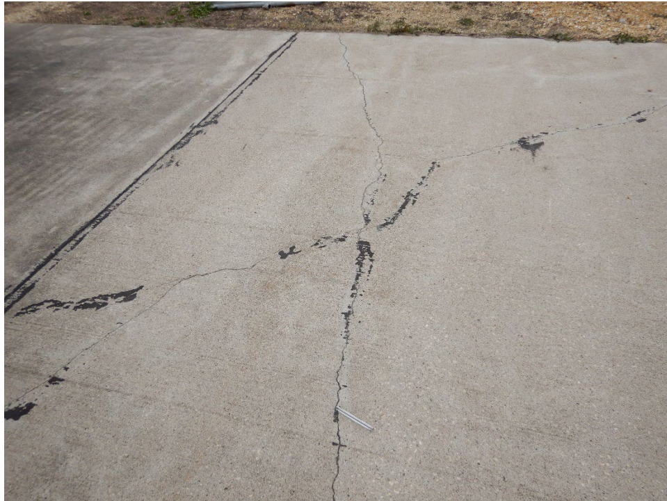
TH01CN-02. Shattered Slab (Sample Unit No. 01).
