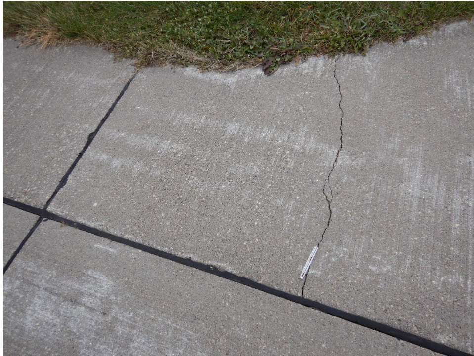
T01CN-02. Corner Break (Sample Unit No. 01).
