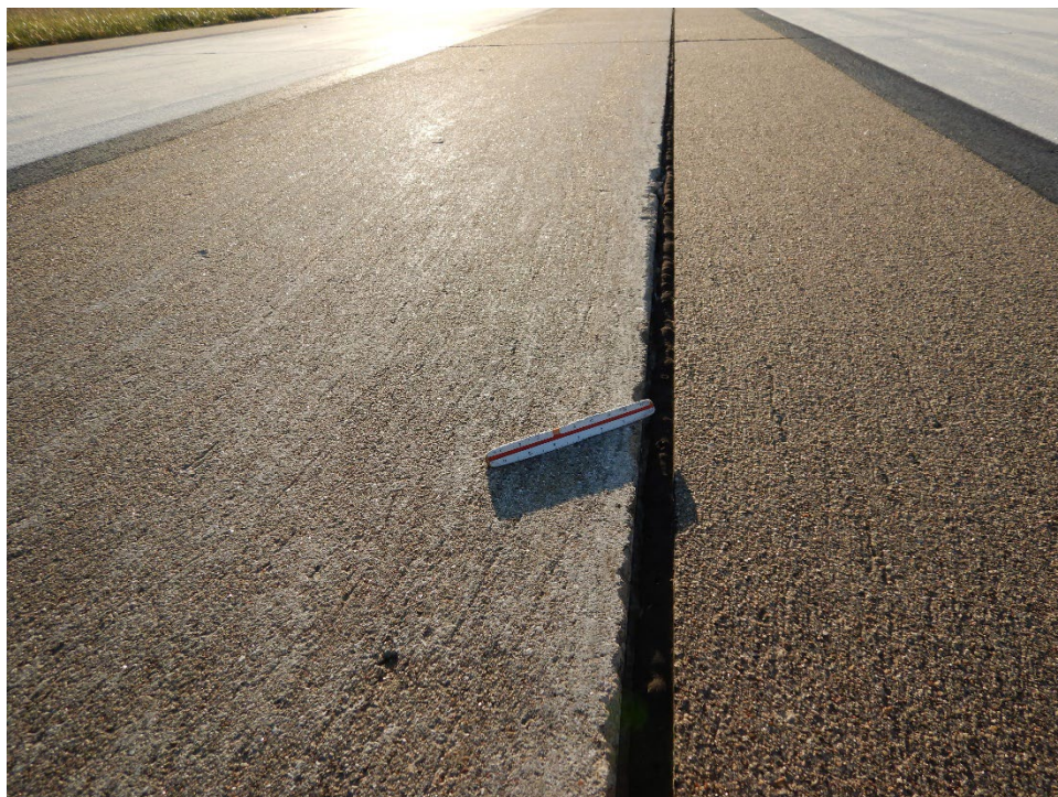
R14CN-01. Faulting (Sample Unit No. 88).
