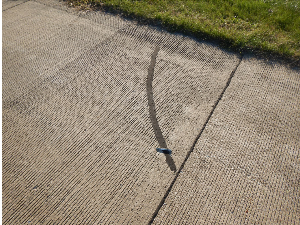
R17FM-01. Corner Break (Sample Unit No. 44).
