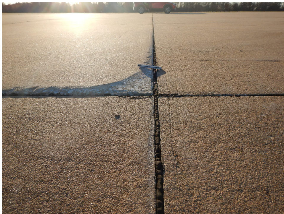
A01FM-02. Faulting (Sample Unit No. 02).
