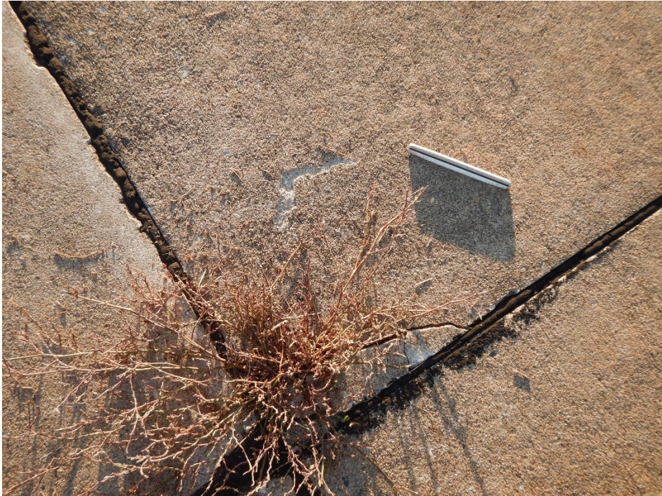
A01FM-01. ASR (Sample Unit No. 07).
