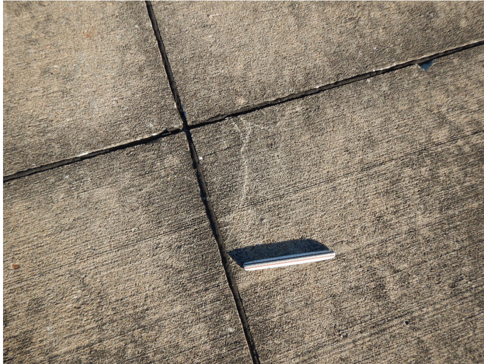
T05FM-01. ASR (Sample Unit No. 05).
