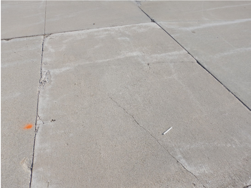
TH01GC-01. Shattered Slab (Sample Unit No. 02).
