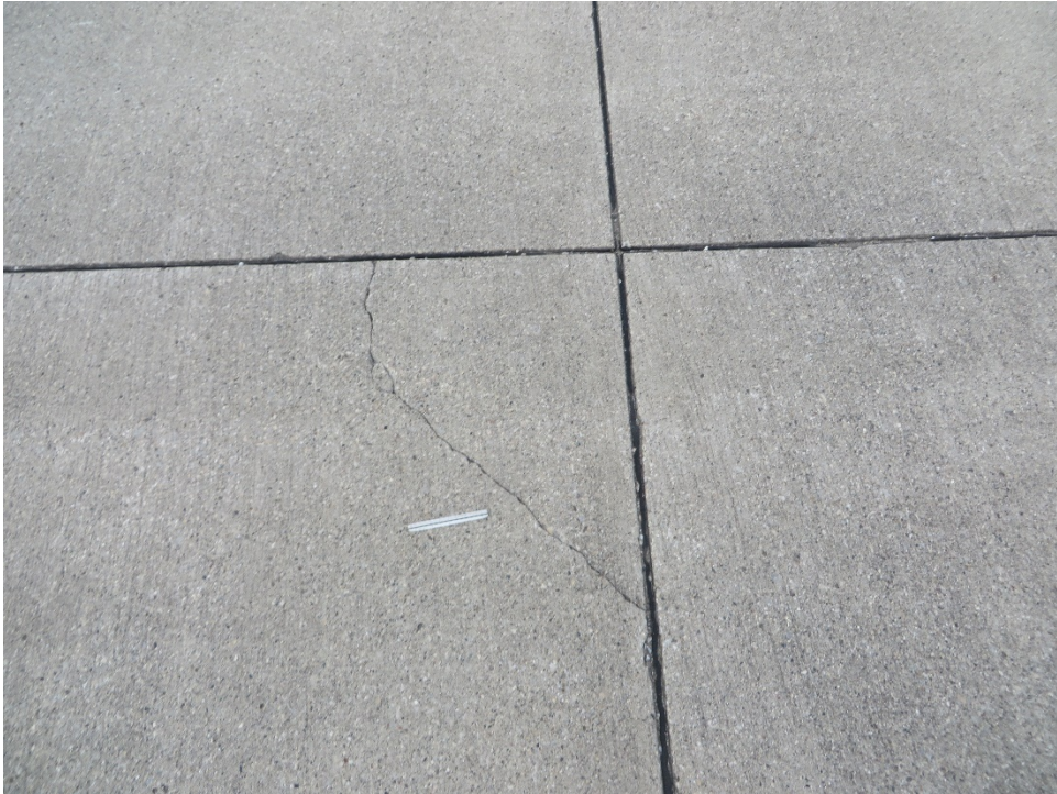
TH01HA-01. Corner Break (Sample Unit No. 01).
