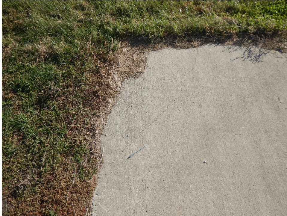
TH01HA-01. Corner Break (Sample Unit No. 08).
