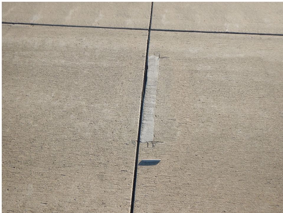
R17HA-01. Small Patching (Sample Unit No. 75).
