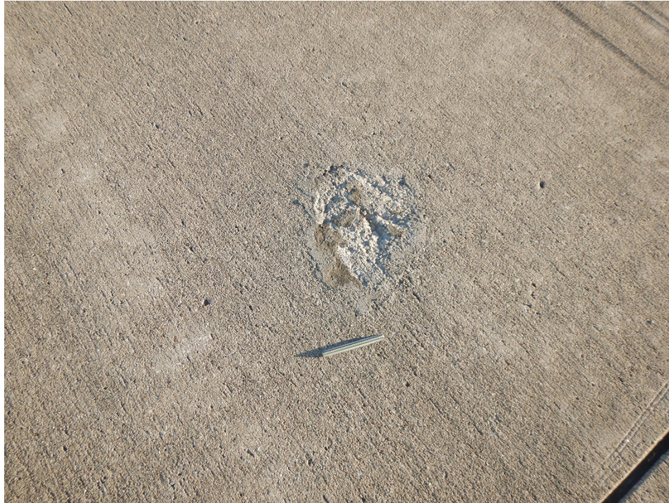
R17HA-01. Scaling (Additional Sample Unit No. 24).
