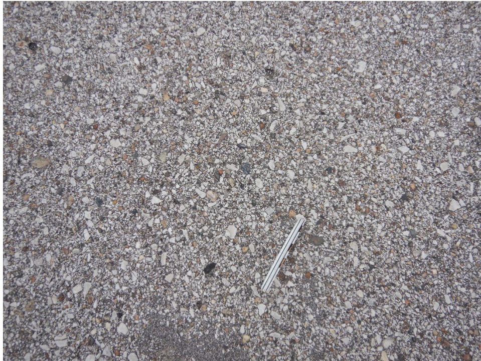
T01HU-01. Weathering (Sample Unit No. 01).
