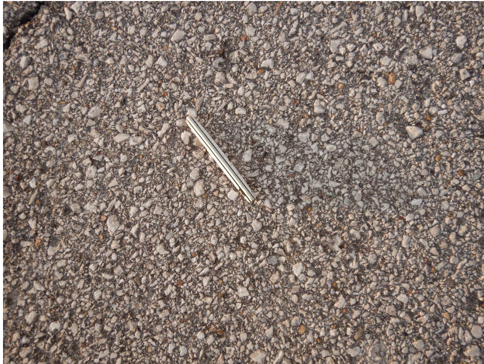
T01IC-04. Weathering (Sample Unit No. 02).
