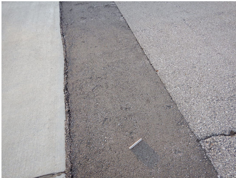
T01IC-04. Patching (Sample Unit No. 02).
