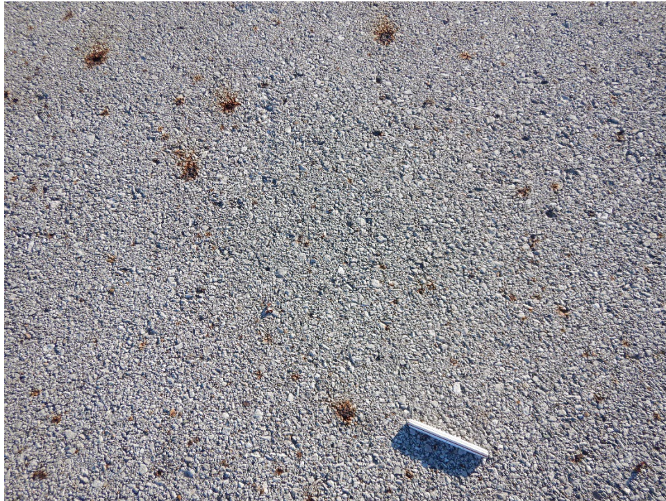
TH01IC-02. Weathering (Sample Unit No. 01).
