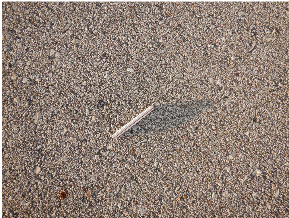
T01IC-01. Weathering (Sample Unit No. 06).
