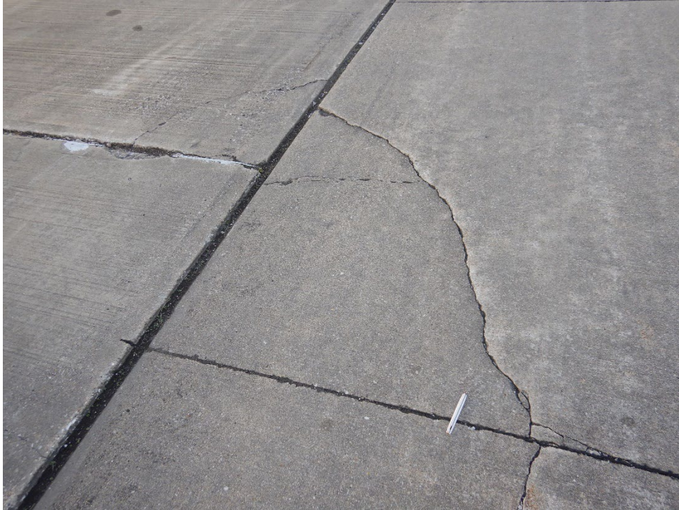
TH02IC-02. Corner Break (Sample Unit No. 13).
