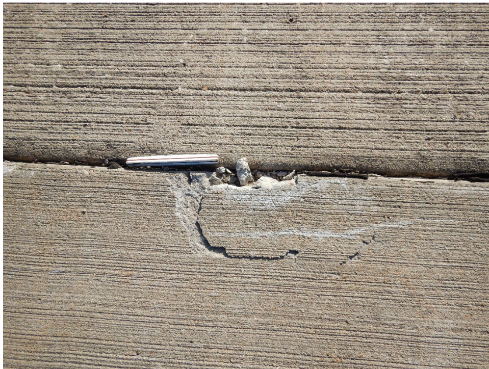
T01IC-06. ASR (Sample Unit No. 01).
