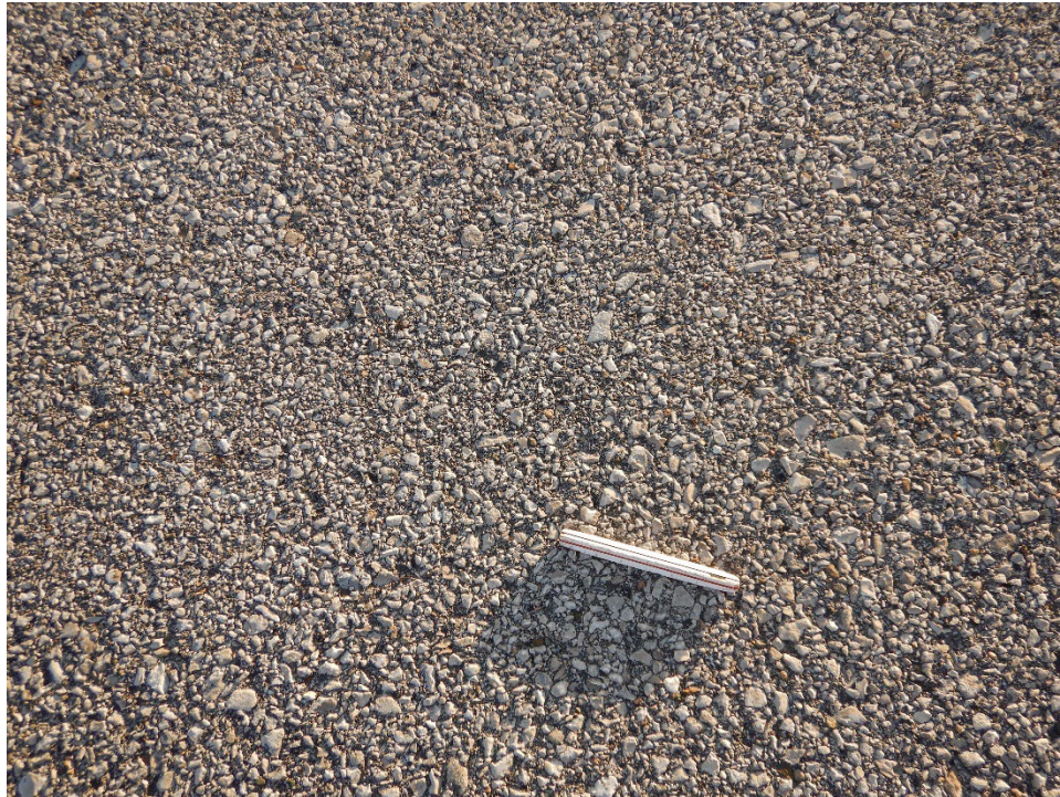
TH02IC-01. Weathering (Sample Unit No. 03).
