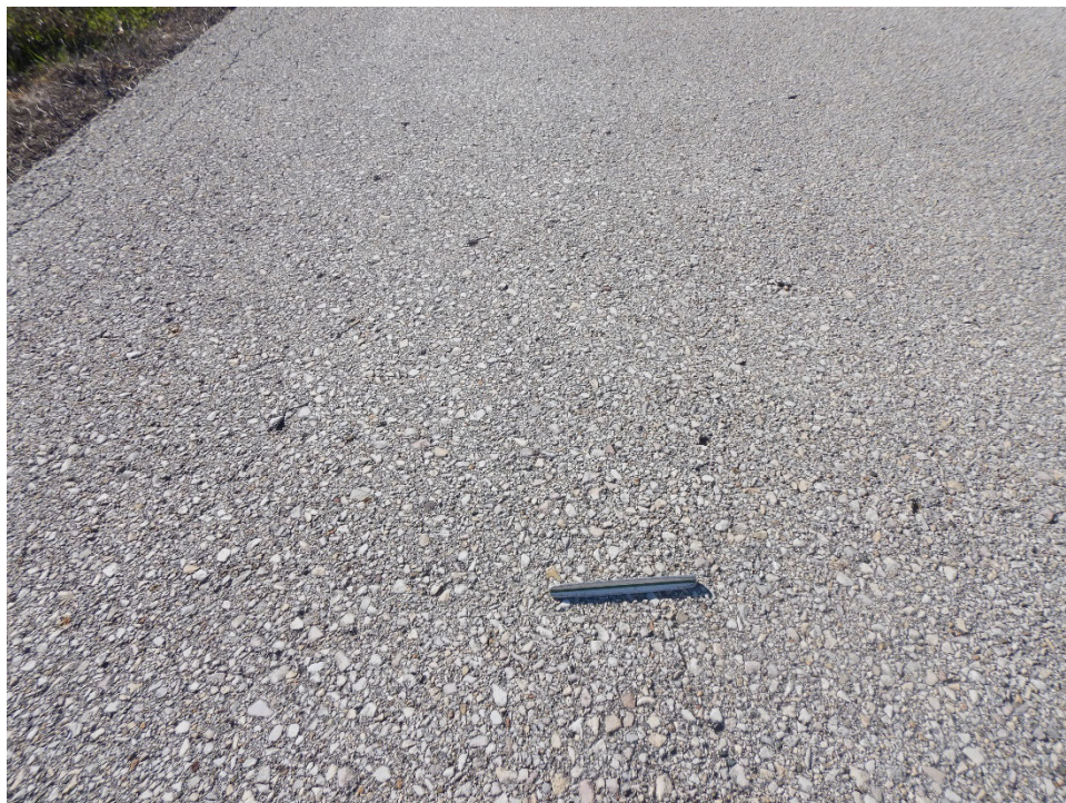
TAIF-01. Raveling (Sample Unit No. 02).
