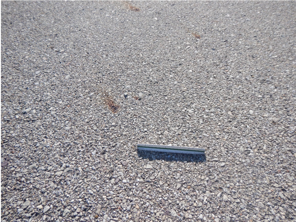
TH01IF-02. Weathering (Sample Unit No. 01).
