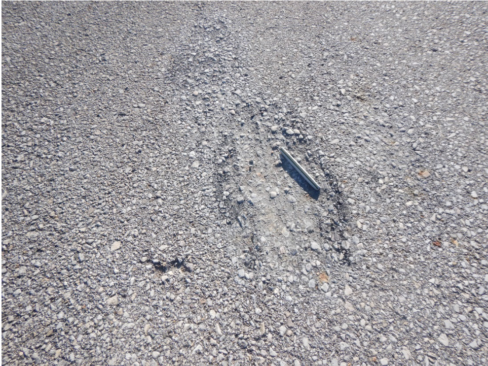
TH01IF-01. Raveling (Sample Unit No. 04).
