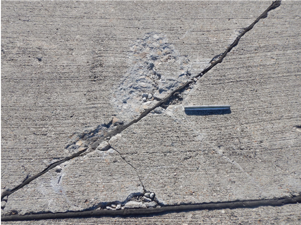
A011F-01. ASR (Sample Unit No. 04).
