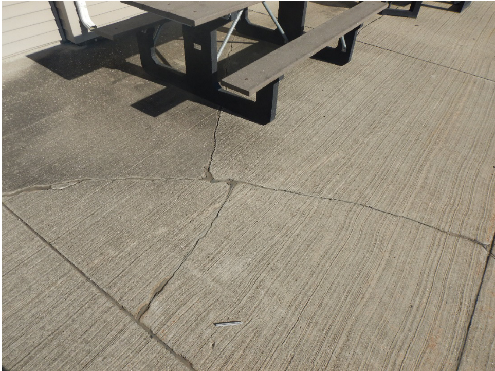
A01IF-01. Shattered Slab (Sample Unit No. 15).
