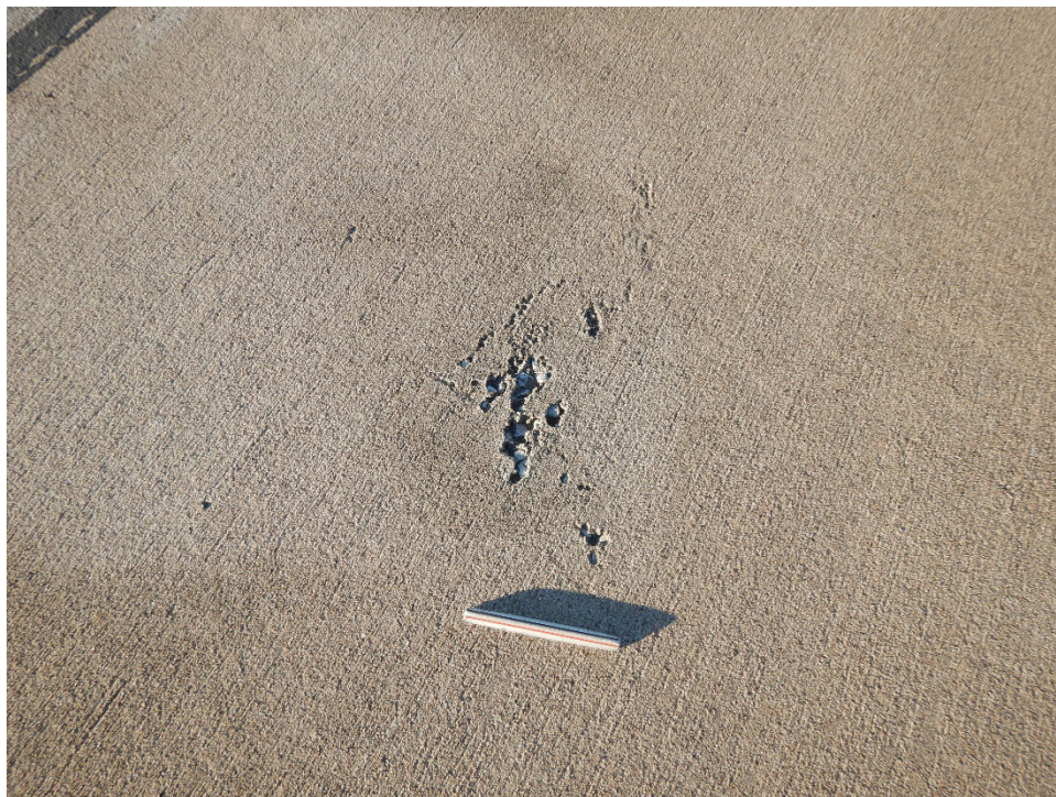
R08KE-01. Scaling (Sample Unit No. 054).
