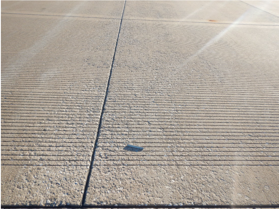
R08KE-01. Scaling (Sample Unit No. 126).
