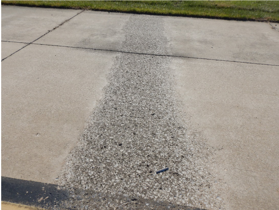
TBKE-01. Scaling (Sample Unit No. 06).
