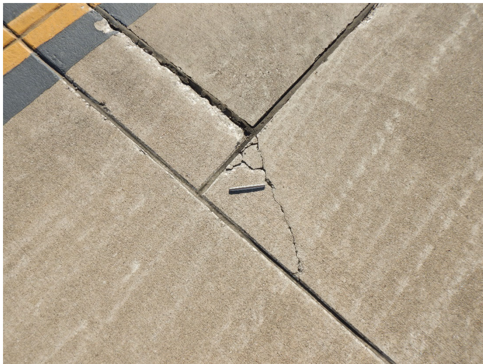
TH01KE-01. Corner Break (Sample Unit No. 24).
