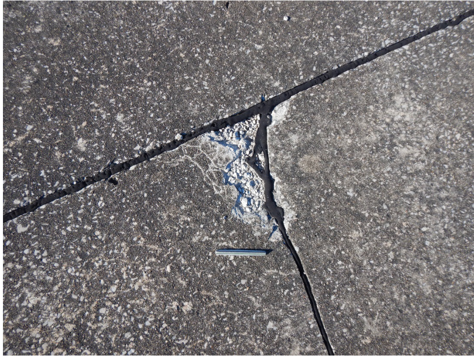
TCKE-02. ASR (Sample Unit No. 09).
