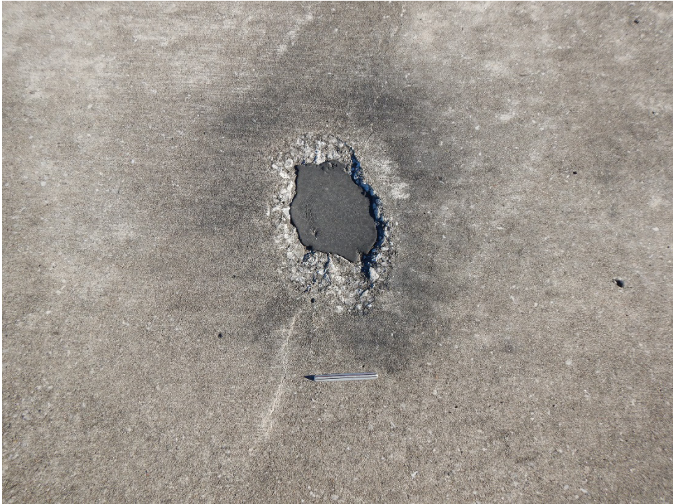
TCKE-02. Small Patching (Sample Unit No. 04).
