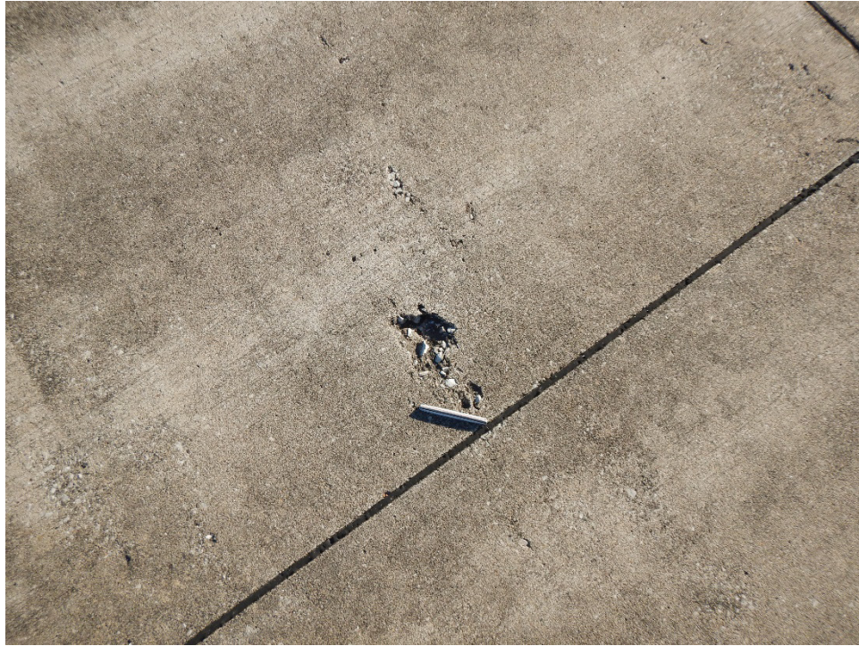
R14KE-02. Scaling (Sample Unit No. 12).
