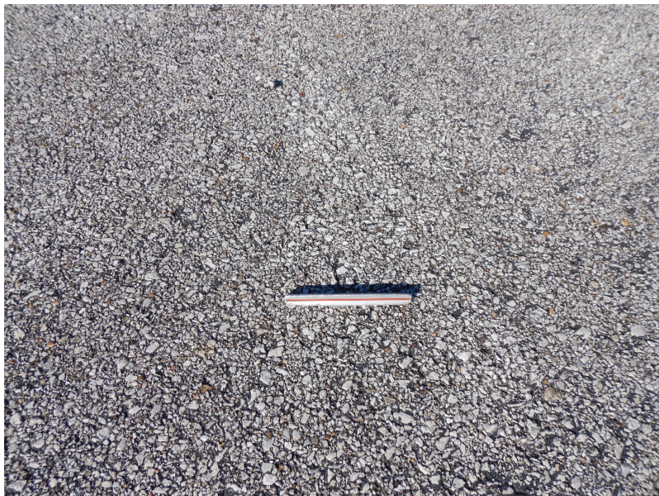
A01KE-02. Weathering (Sample Unit No. 08).
