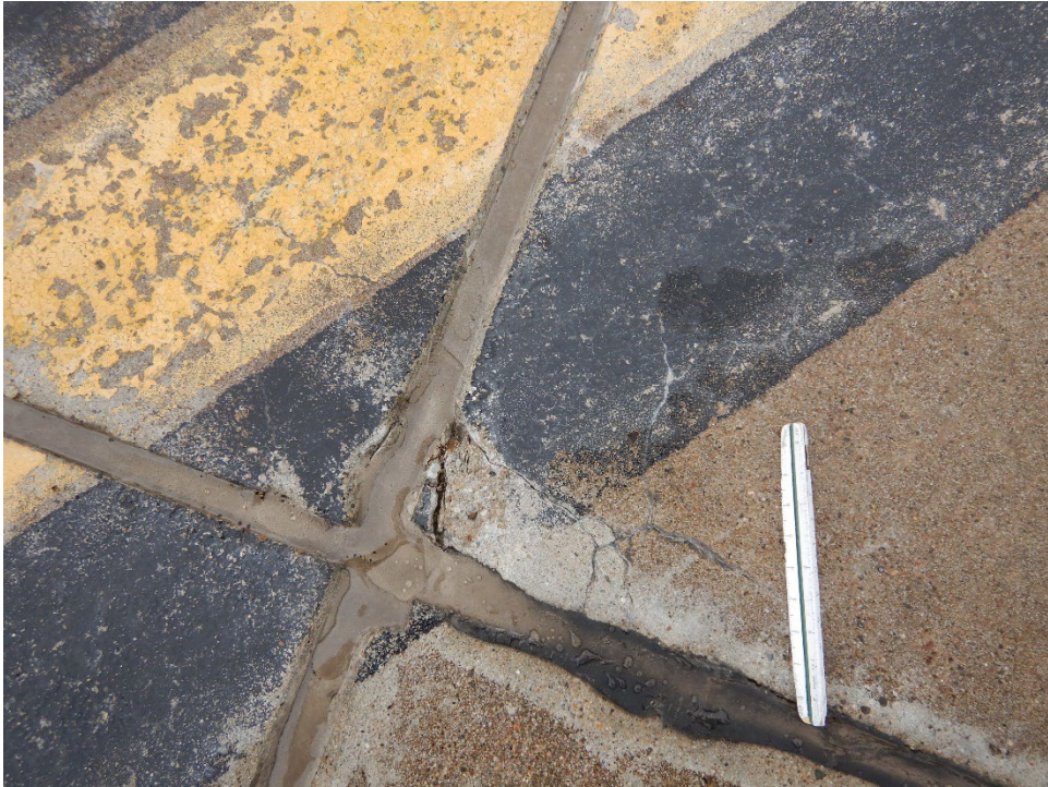
T02KN-01. ASR (Sample Unit No. 06).
