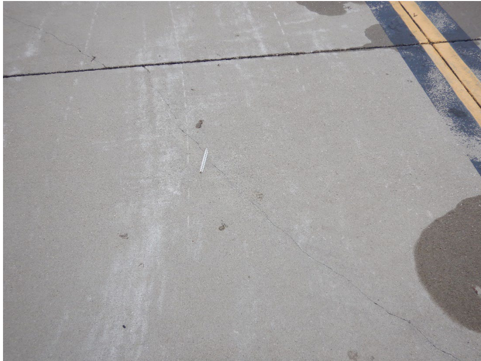
TH01KN-02. Corner Break (Sample Unit No. 01).
