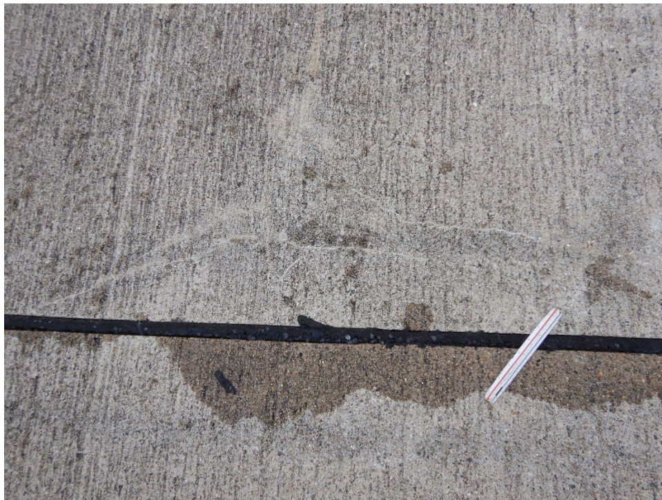
T03KN-02. ASR (Sample Unit No. 15).
