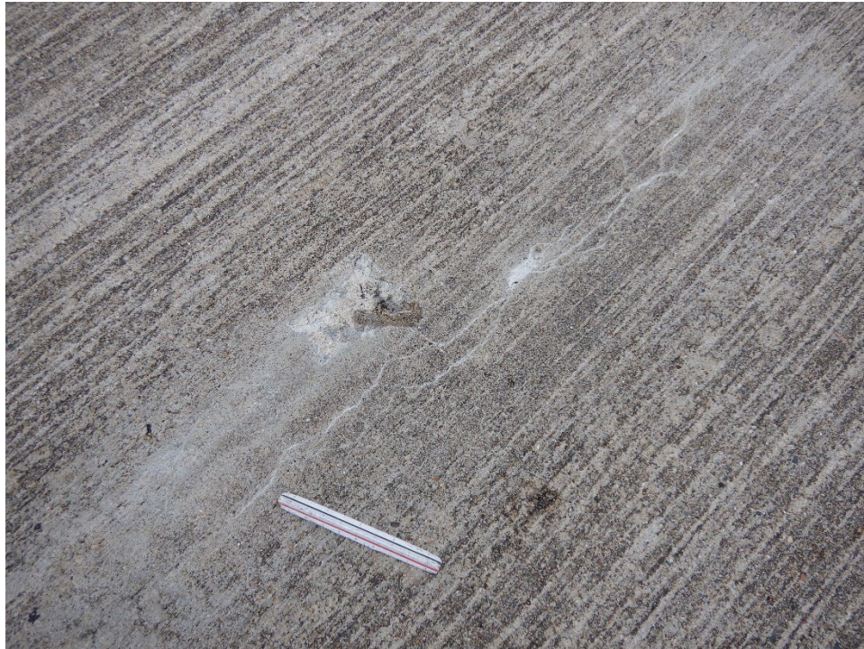
T03KN-02. ASR (Sample Unit No. 05).
