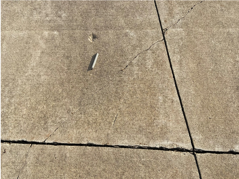
T04MQ-01. Corner Break (Sample Unit No. 01).
