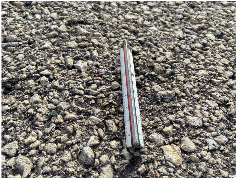
T02MQ-02. Weathering (Sample Unit No. 01) (1).
