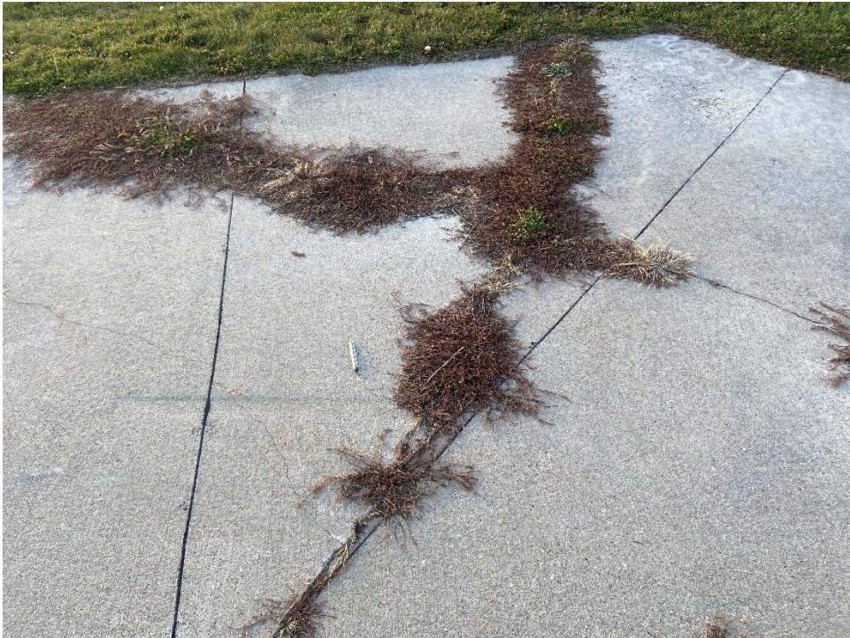
TH01MQ-03. Shattered Slab (Sample Unit No. 01).
