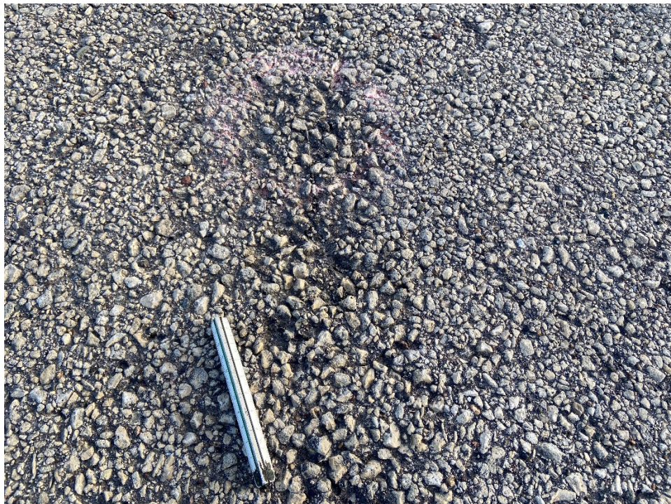
T03MQ-01. Weathering (Sample Unit No. 01).
