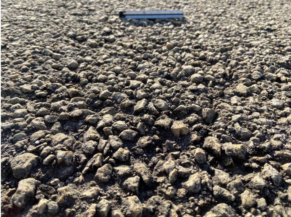
T02MQ-02. Weathering (Sample Unit No. 01) (2).
