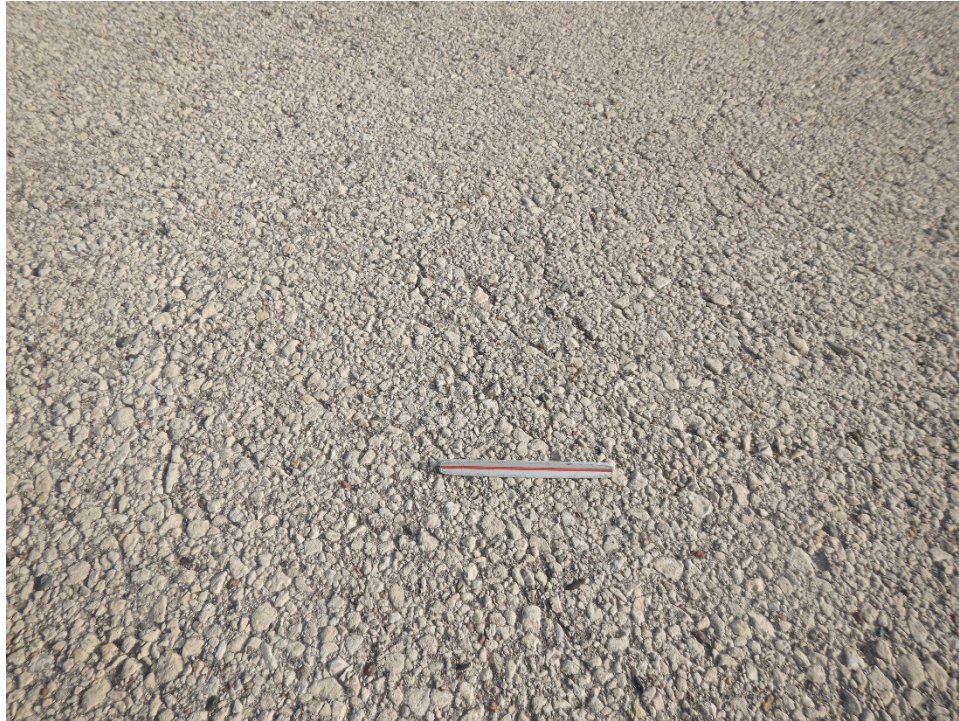
T03MQ-01. Weathering (Sample Unit No. 01).
