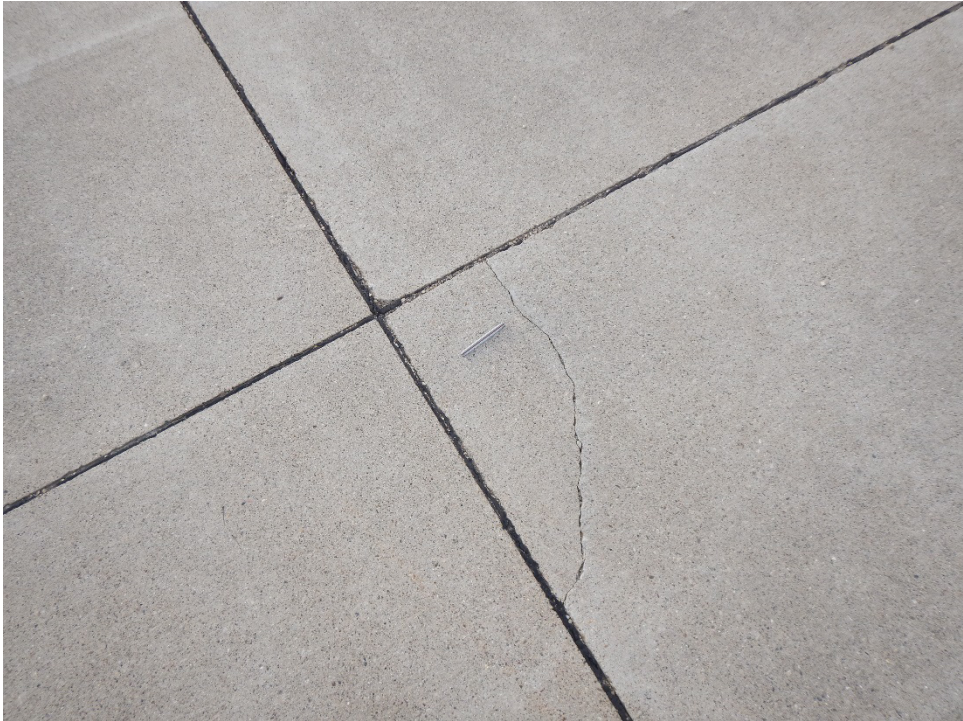
A01MQ-01. Corner Break (Sample Unit No. 09).
