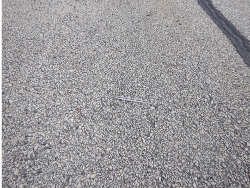
TAMQ-02. Weathering (Sample Unit No. 01).
