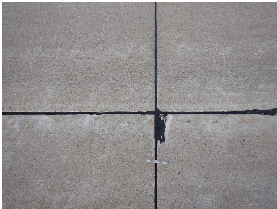
R15MQ-01. Joint Spalling (Sample Unit No. 33).
