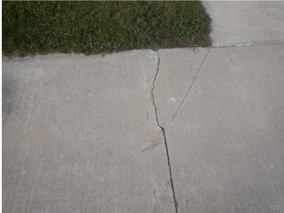
TH01MQ-02. Corner Break (Sample Unit No. 01).
