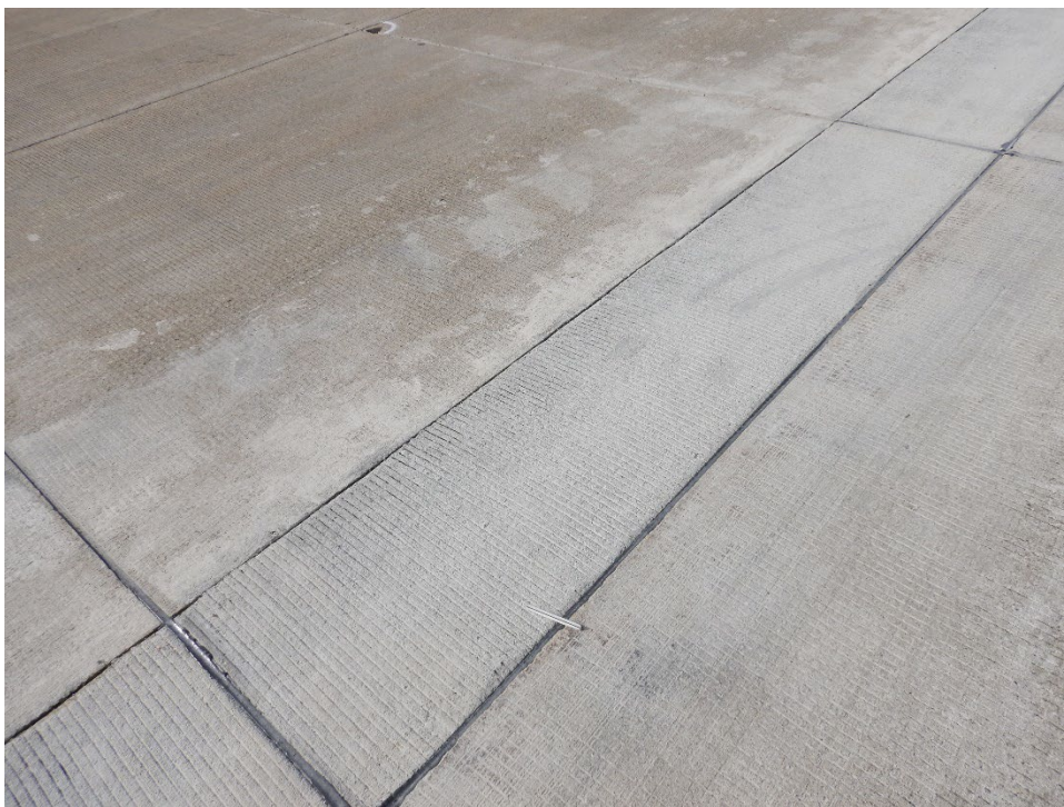
R13OE-01. Large Patching (Sample Unit No. 44).
