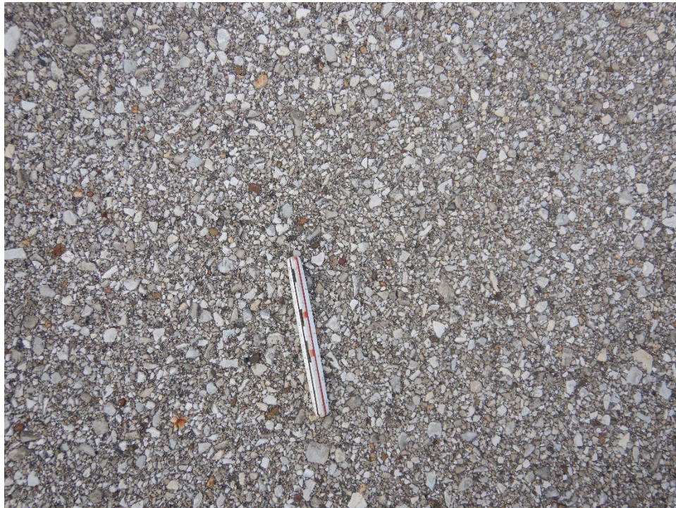
TH01OE-01. Weathering (Sample Unit No. 02).
