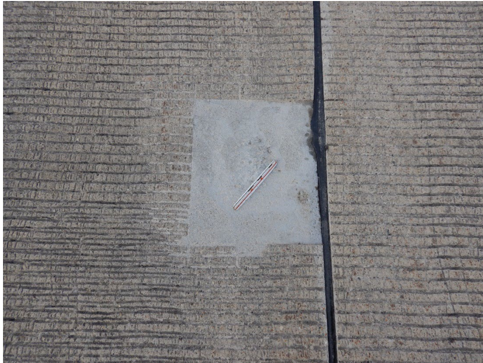
R13OE-01. Small Patching (Sample Unit No. 08).
