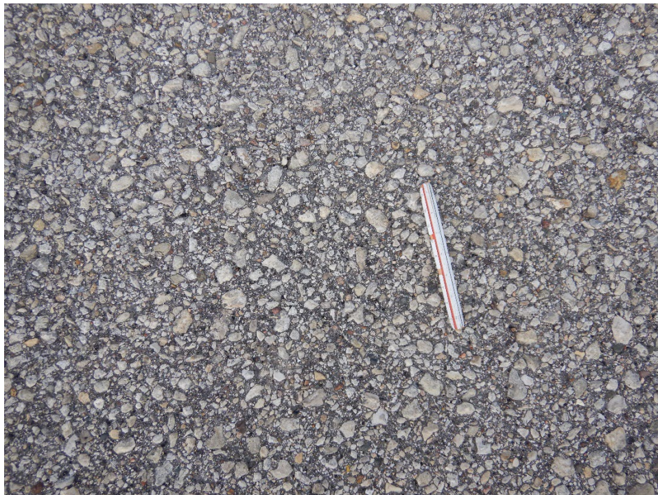
TH01OE-02. Weathering (Sample Unit No. 02).
