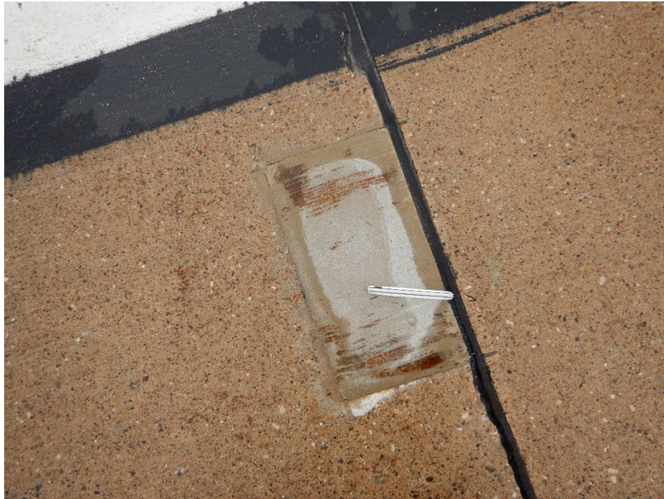
R16PE-03. Small Patching (Sample Unit No. 34).
