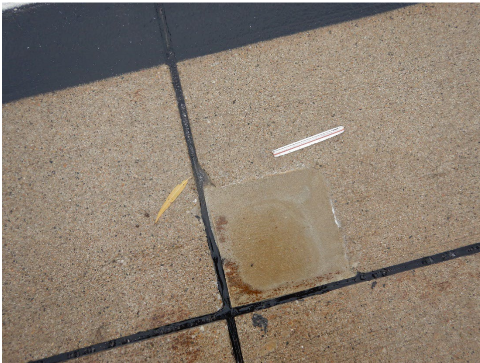
R16PE-07. Small Patching (Sample Unit No. 12).
