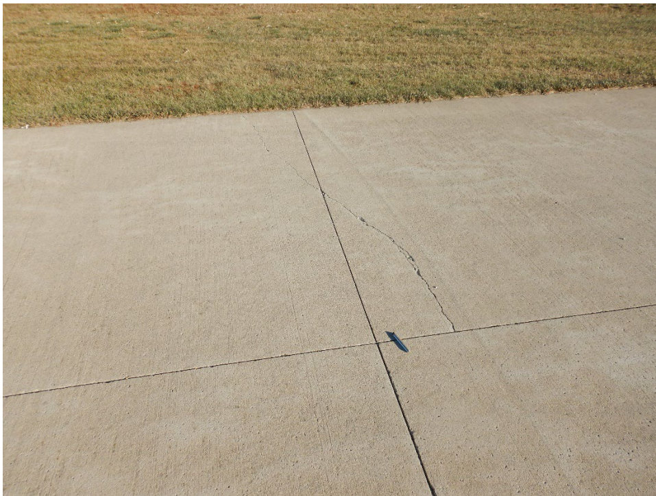
TH01PO-01. Corner Break (Sample Unit No. 03).
