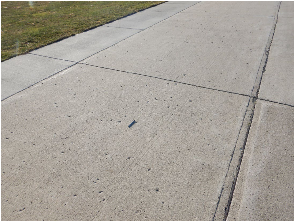
TH01PO-03. Popouts (Sample Unit No. 01).
