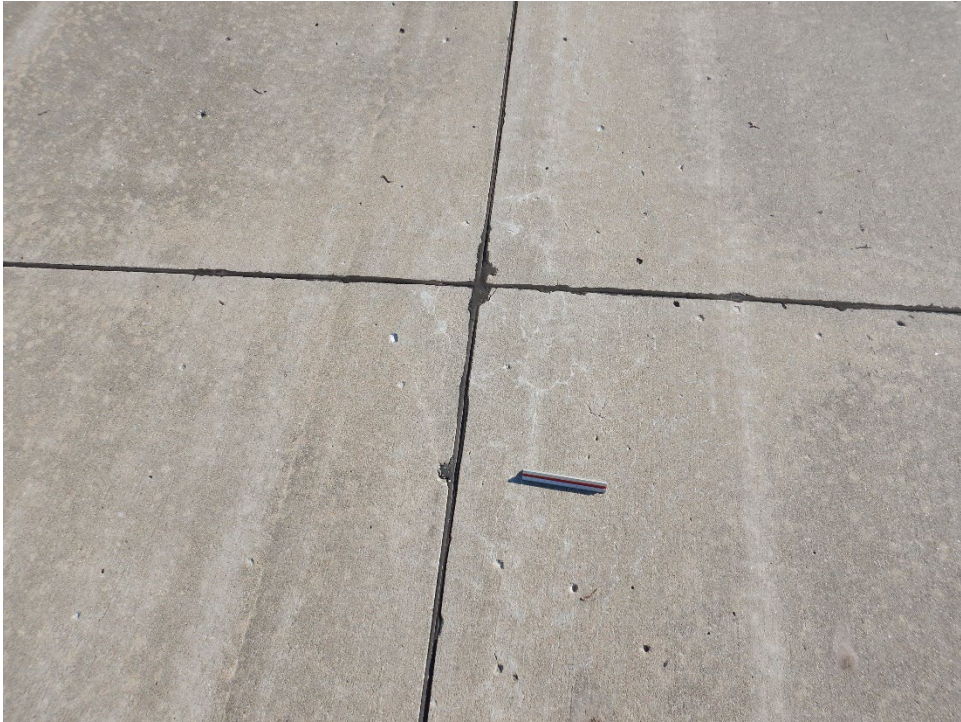
T01RO-01. ASR (Sample Unit No. 17).
