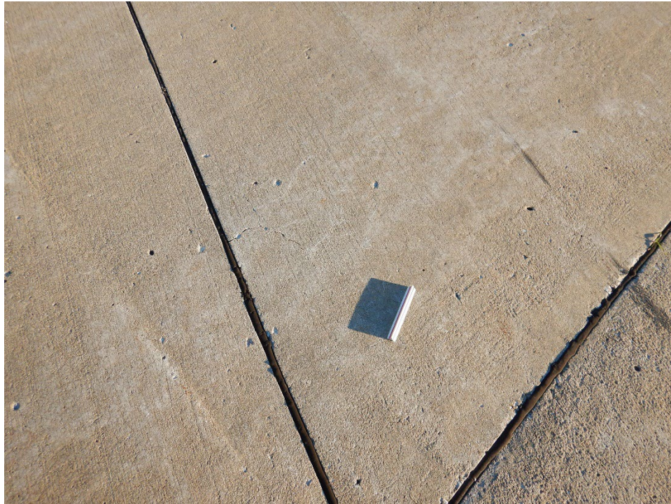
R17RO-04. ASR (Sample Unit No. 02).
