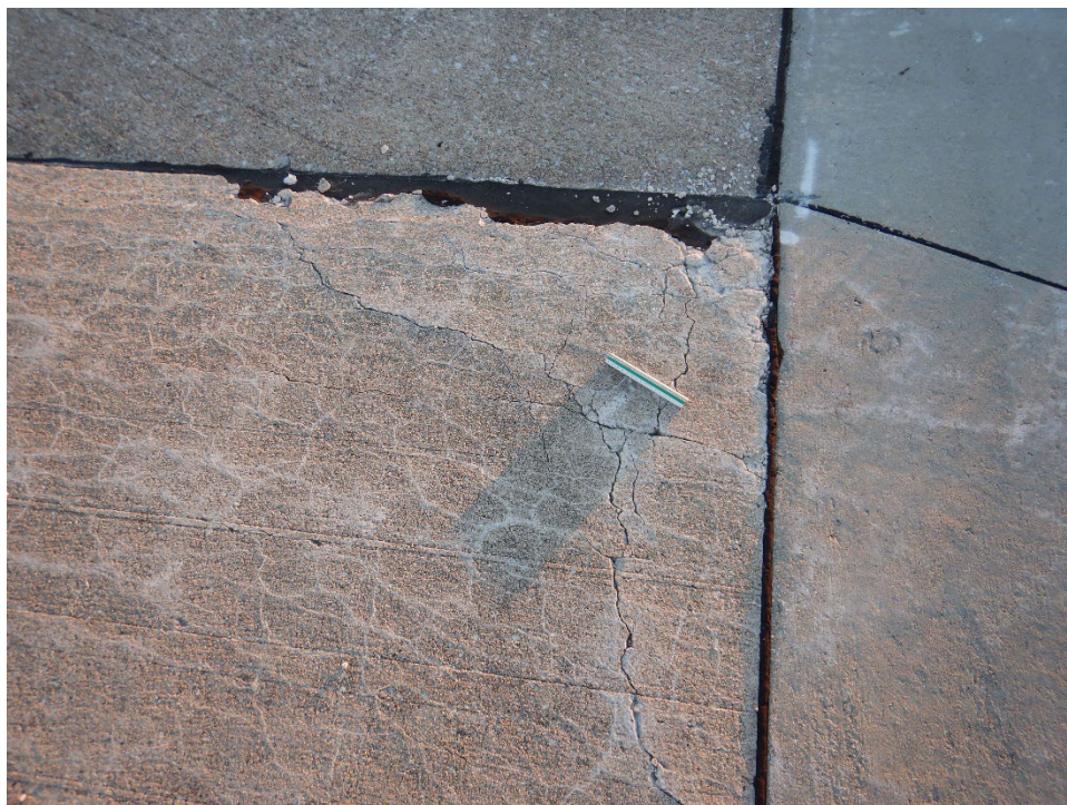
R17RO-02. ASR (Sample Unit No. 02).
