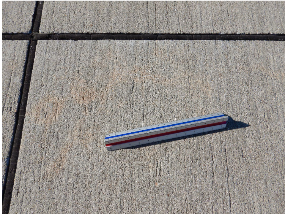
T05RO-01. ASR (Sample Unit No. 28).
