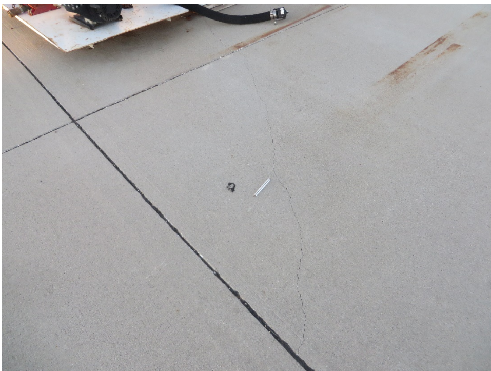
A01RC-01. Corner Break (Sample Unit No. 04).
