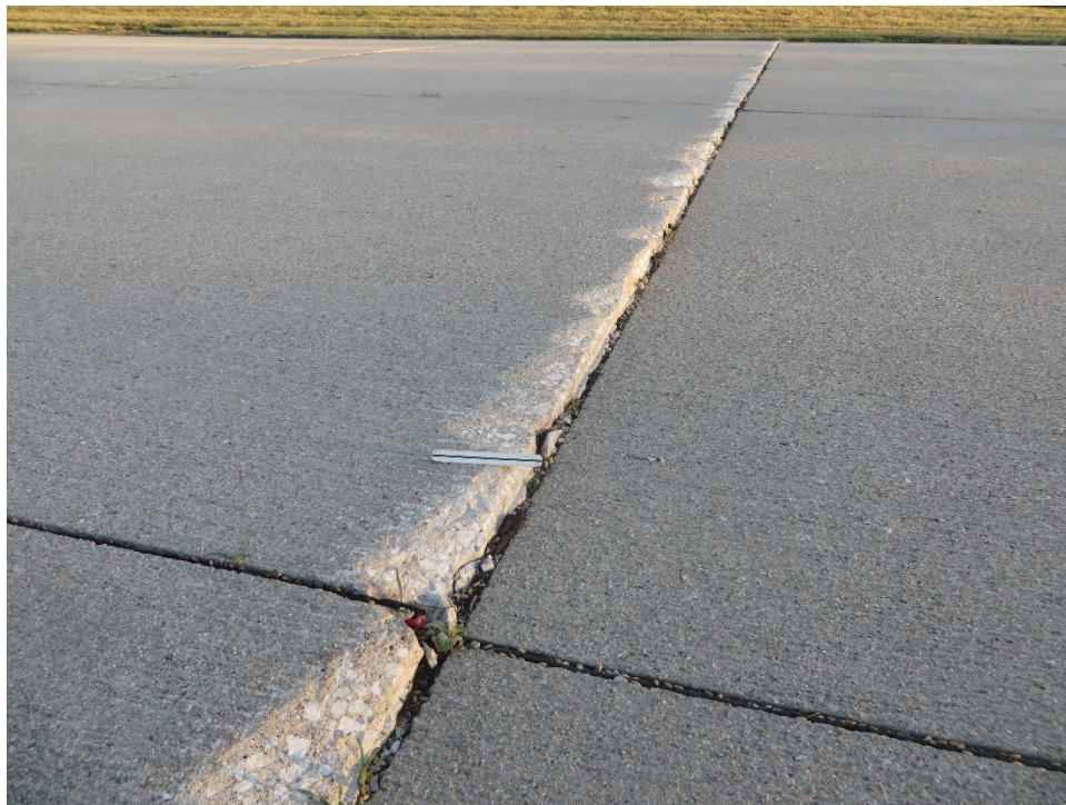
A02RC-01. Faulting (Sample Unit No. 11).
