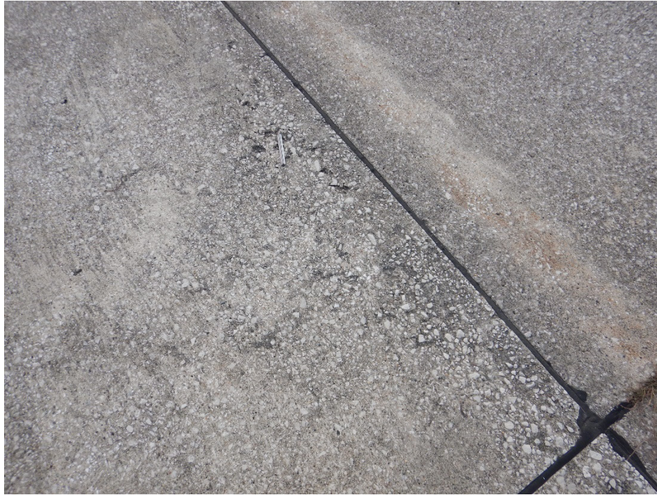
R12RC-01. Scaling (Sample Unit No. 15).
