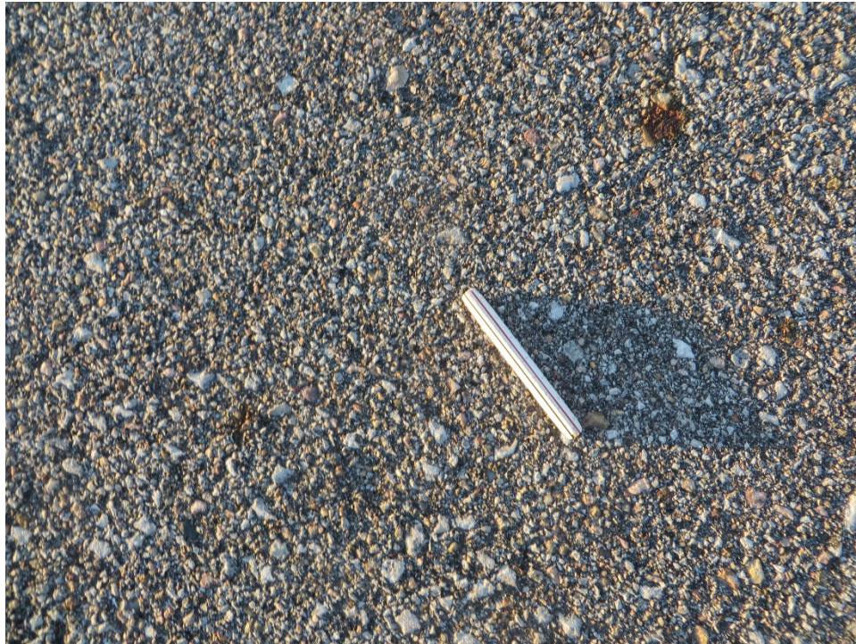
TH01SH-01. Weathering (Sample Unit No. 01).
