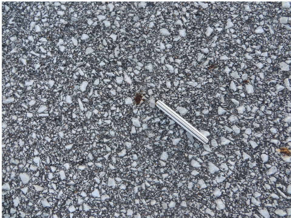
TH01SH-03. Weathering (Sample Unit No. 01).
