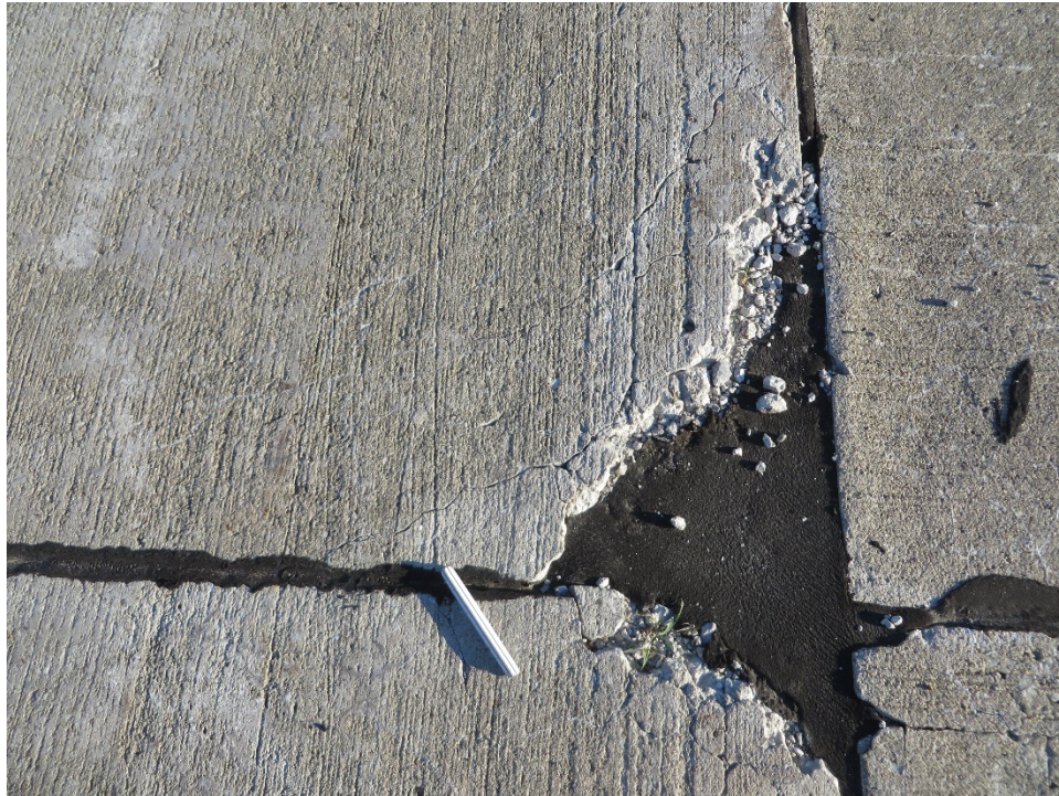
T02SH-01. ASR (Sample Unit No. 03).
