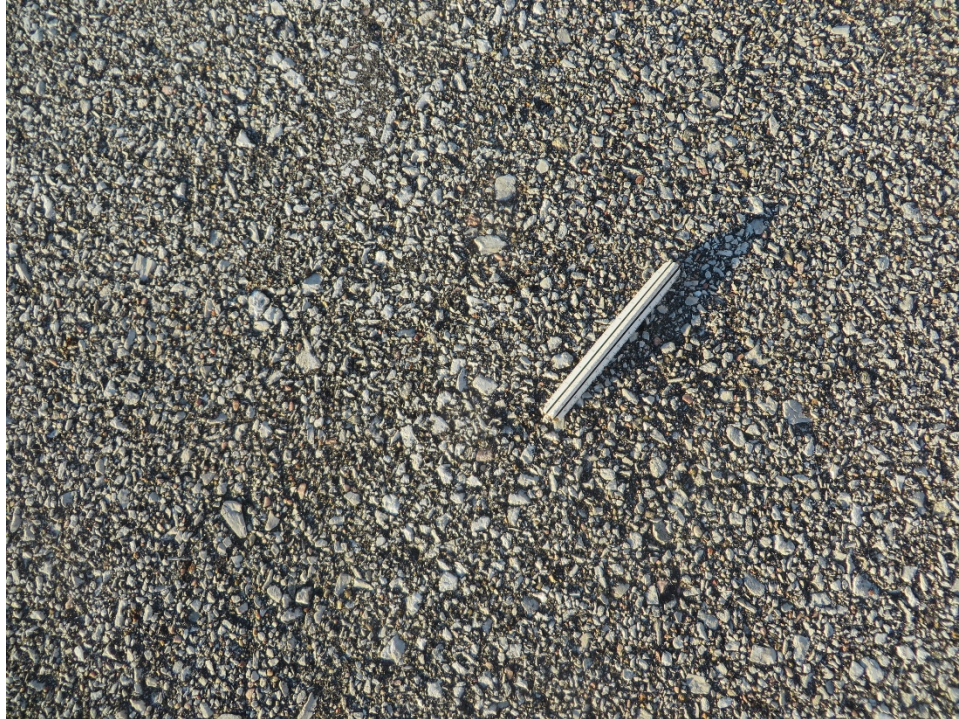
TH01SH-04. Weathering (Sample Unit No. 01).
