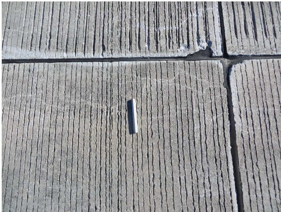
R04SH-02. ASR (Sample Unit No. 08).
