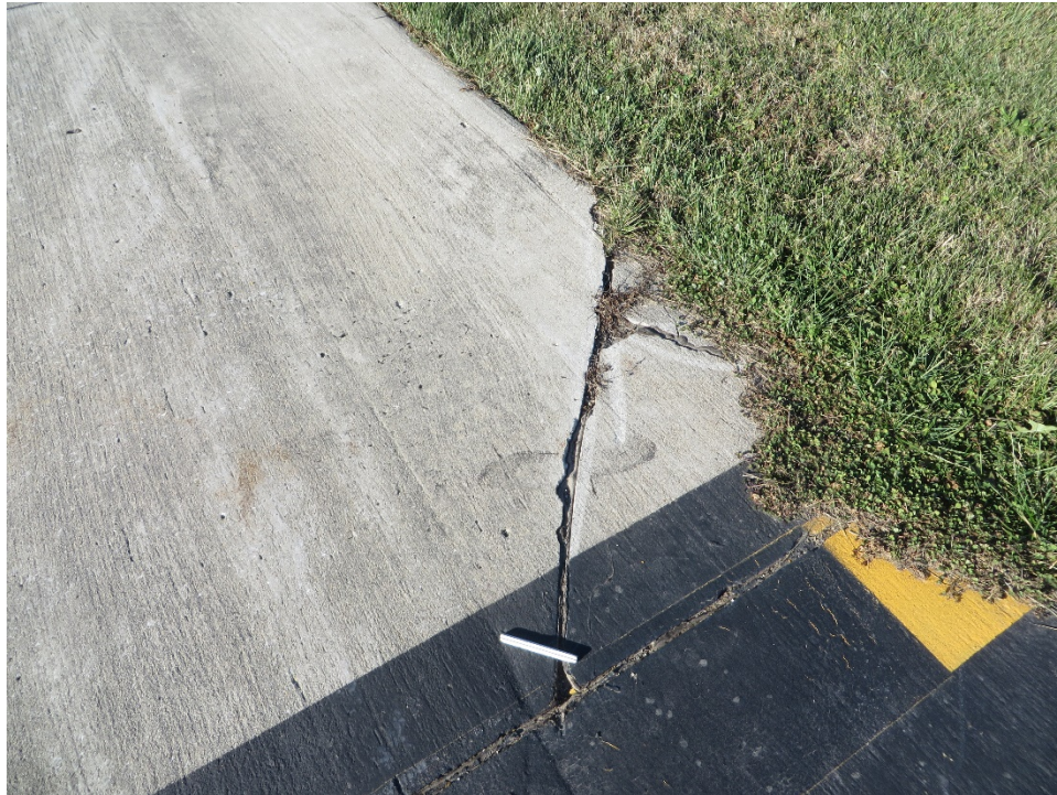
T03SH-03. Corner Break (Sample Unit No. 02).
