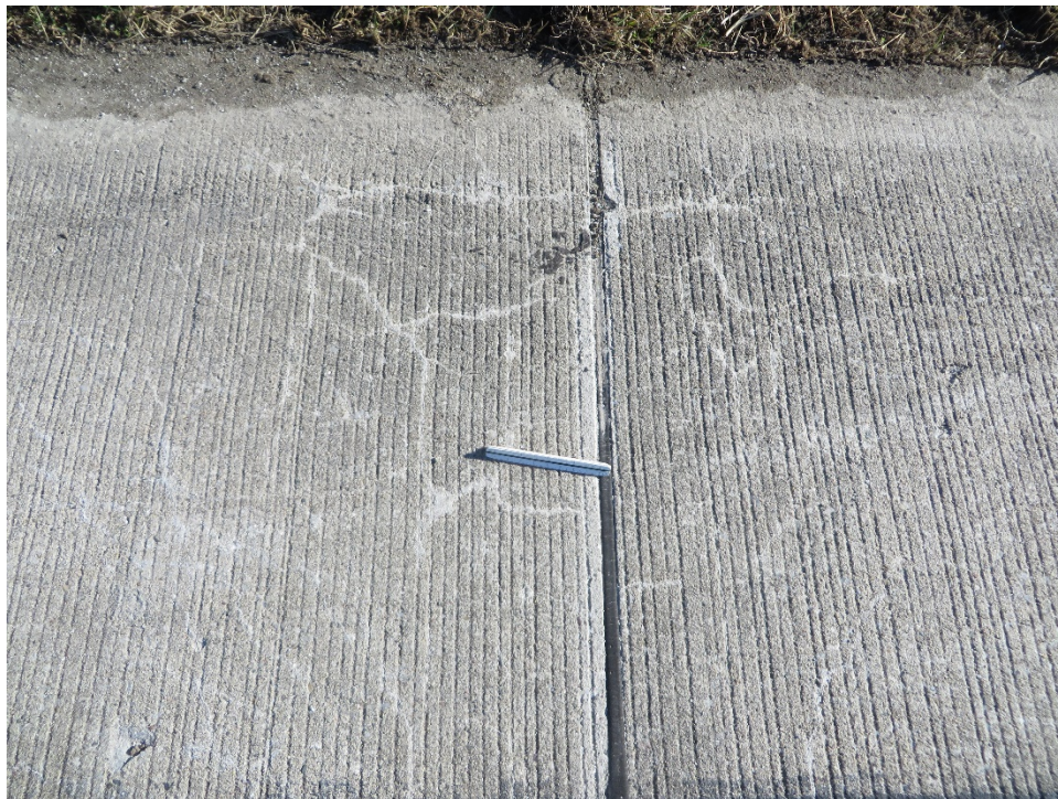
R04SH-01. ASR (Sample Unit No. 07).
