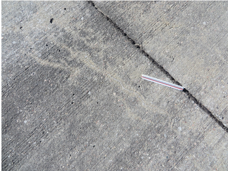
R12SH-01. ASR (Sample Unit No. 55).
