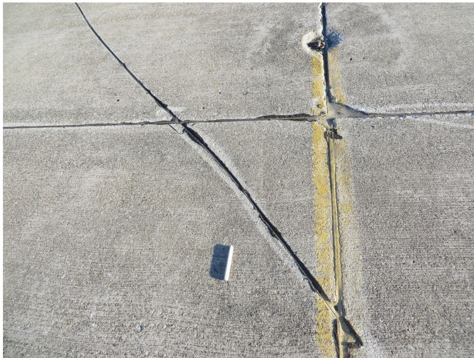
A02SH-01. Corner Break (Sample Unit No. 03).
