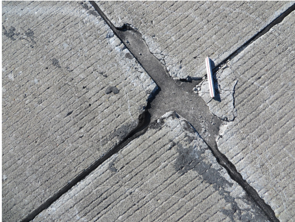
R04SH-02. ASR (Sample Unit No. 17).
