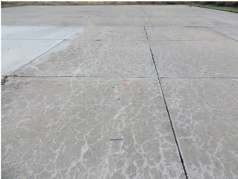
T04SH-01. ASR (Sample Unit No. 03).
