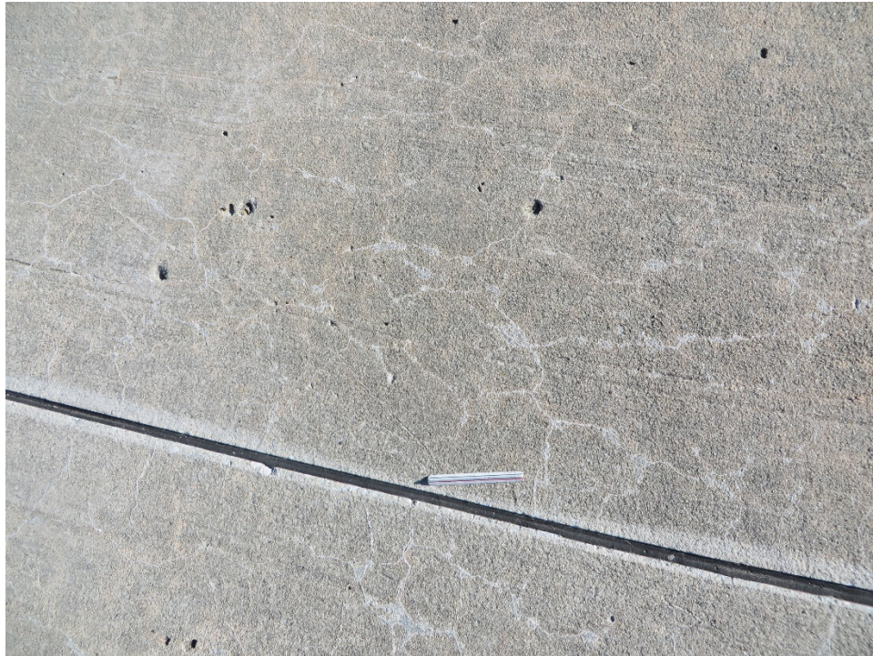
T04SH-01. ASR (Sample Unit No. 07).
