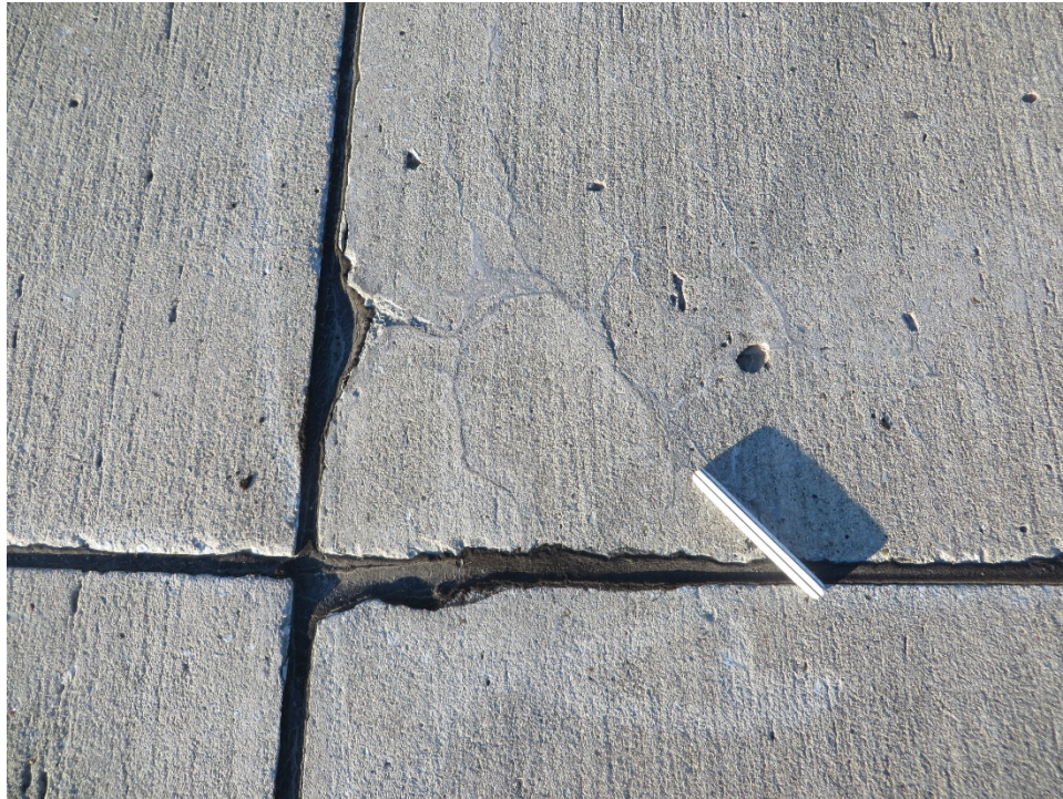
A02SH-02. ASR (Sample Unit No. 04).
