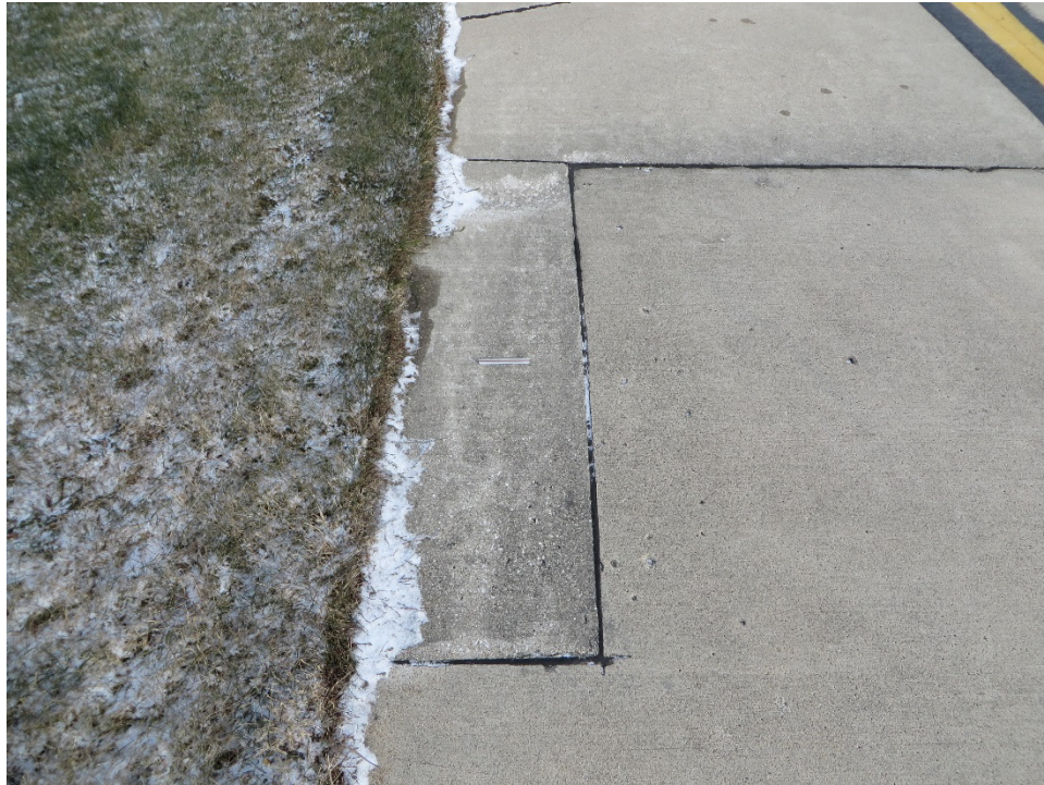
T03IS-02. Large Patching (Sample Unit No. 01).
