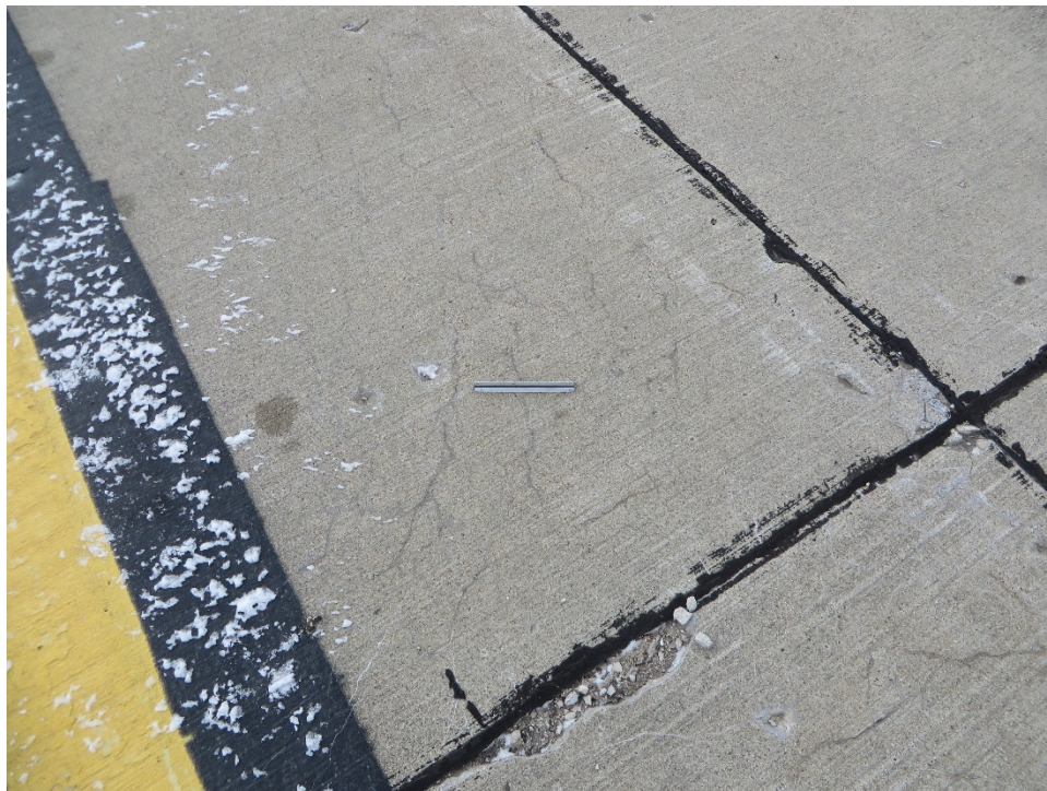
T04IS-01. ASR (Sample Unit No. 05).
