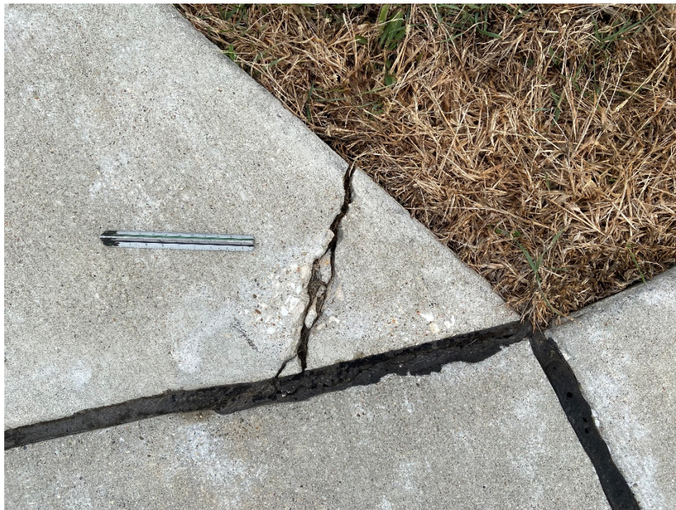
T01WU-01. Corner Break (Sample Unit No. 01).
