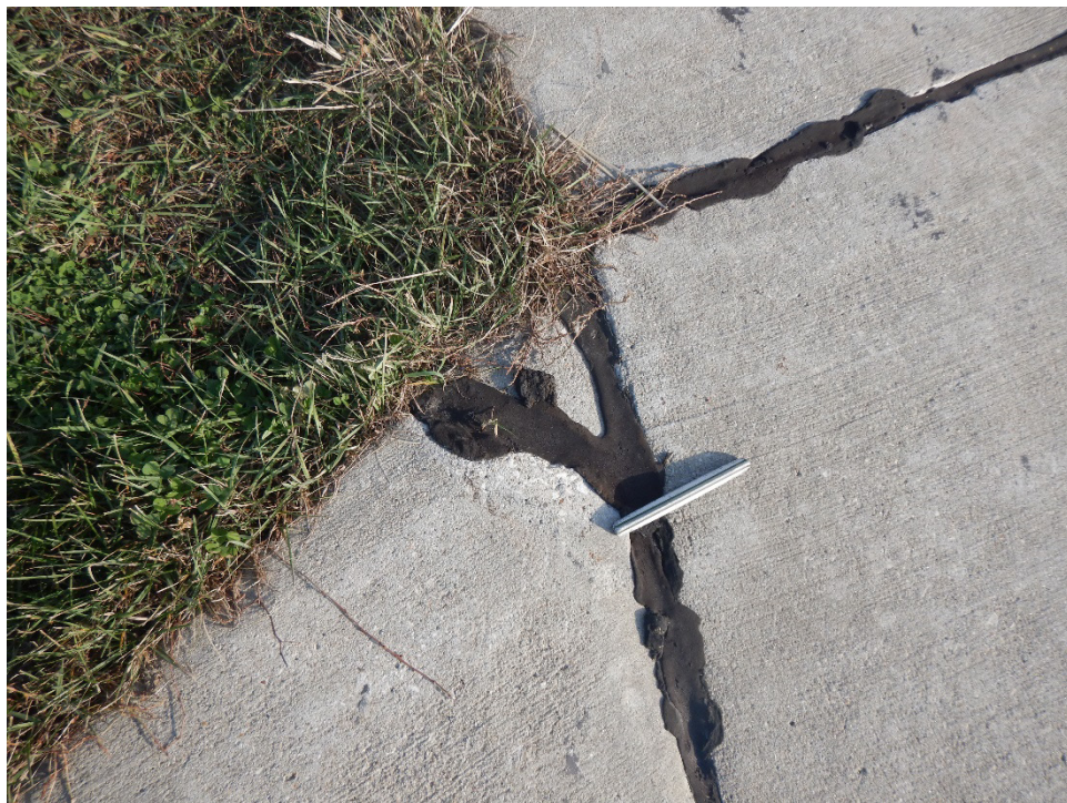
T01WU-01. Corner Break (Sample Unit No. 01).
