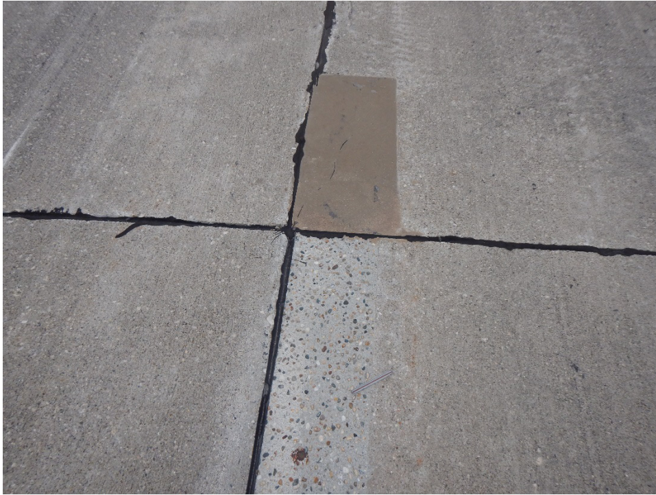
R17WU-01. Small Patching (Sample Unit No. 04).
