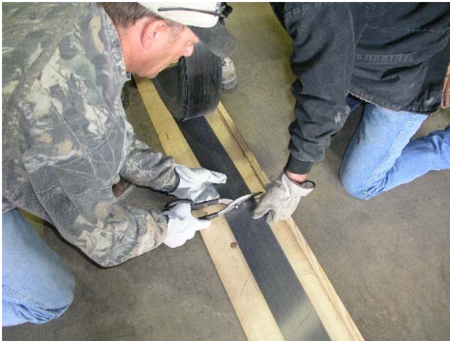
Figure 16. Cutting the CFRP plates.
