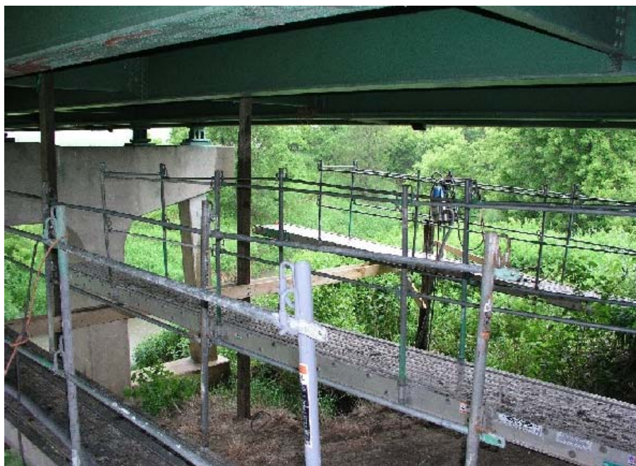
Figure 9. Temporary work scaffolding.
