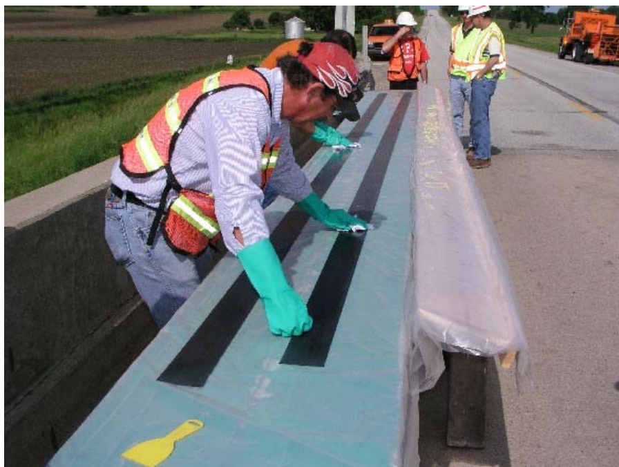
Figure 13. Cleaning the CFRP plate bonding surface.
