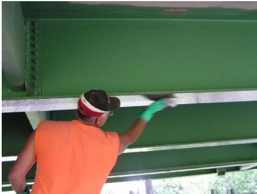
Figure 12. Cleaning the girder surface after sandblasting.
