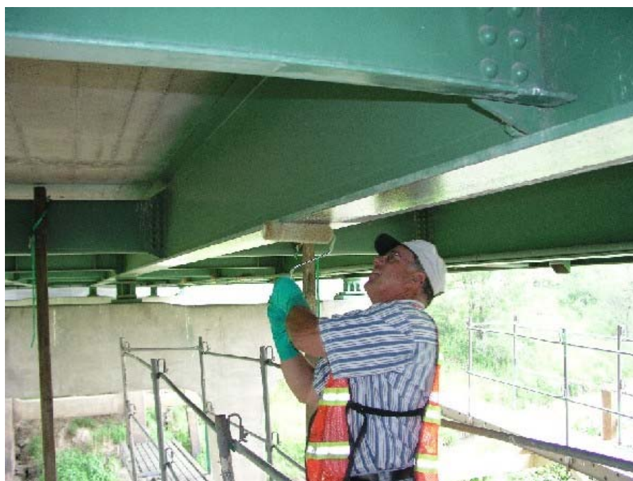
Figure 14. Applying FRS 1000 Primer to bottom girder flange.
