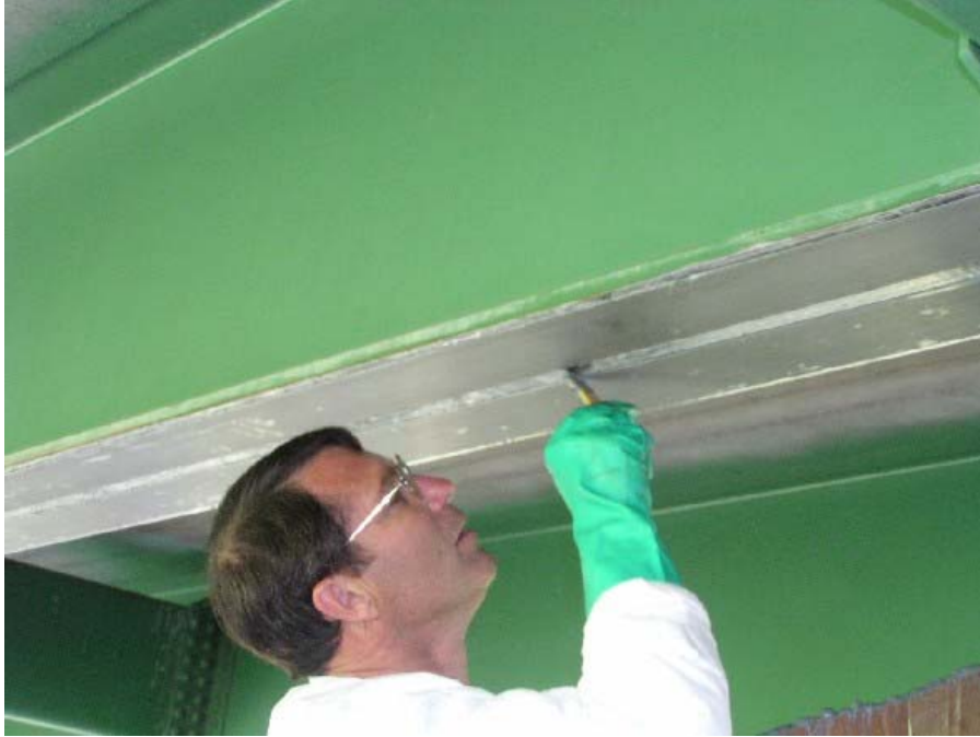
Figure 20. Removal of excess epoxy.
