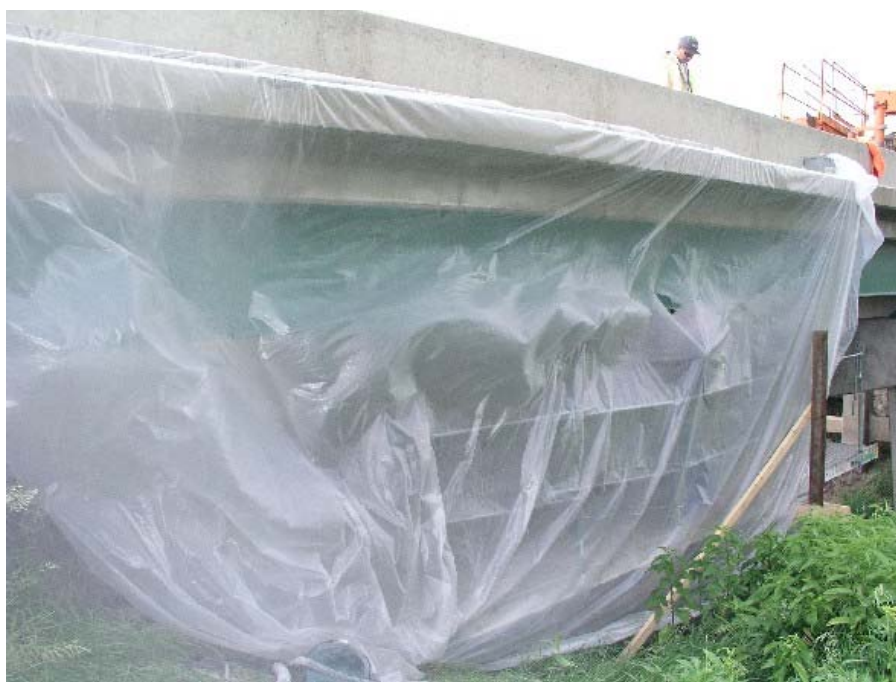
Figure 10. Confinement of work area during sandblasting.
