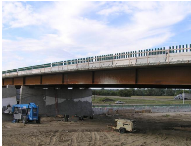
Figure 1. Bridge Pier and Girders during Phase I construction
