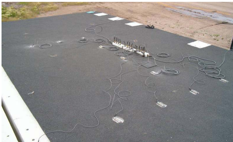
Figure 18. Top of Deck Test Instrumentation, strain gage cluster.
