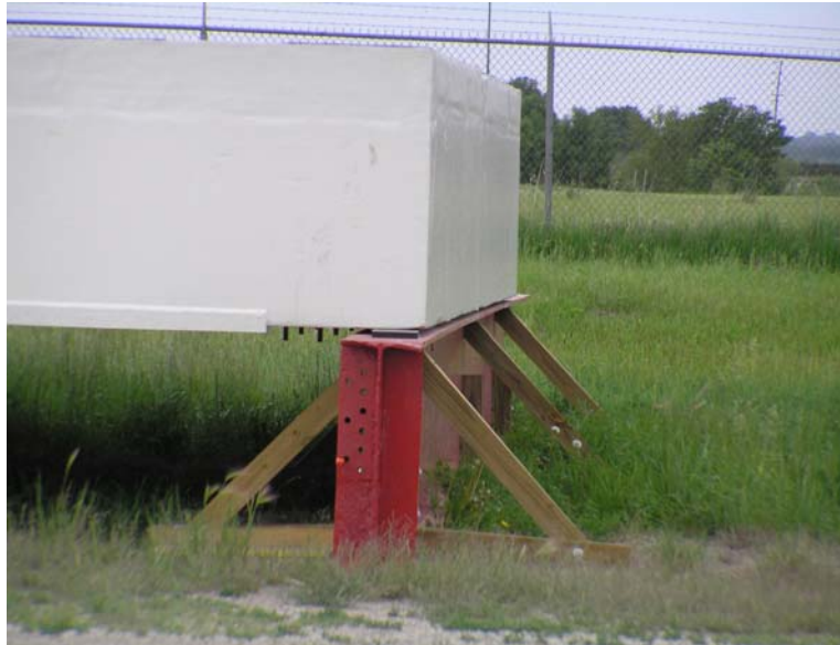
Figure 12. Temporary abutments for Iowa DOT composite bridge.
