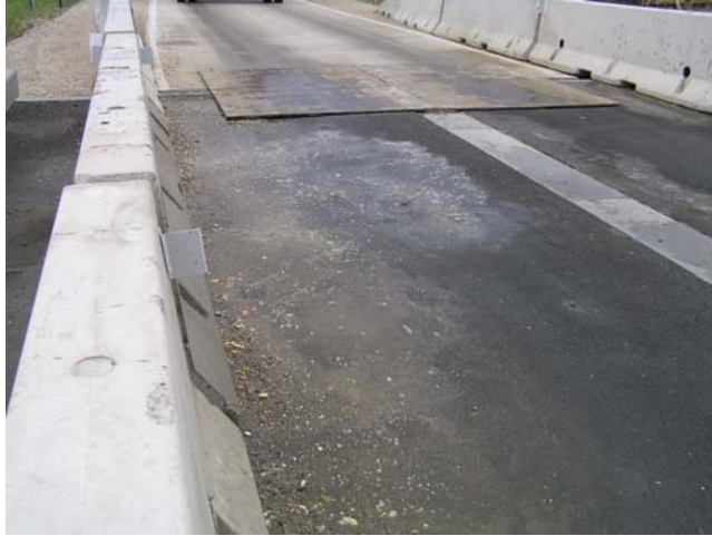
Figure 33. Jersey barrier and steel plate on FRP Bypass Bridge.
