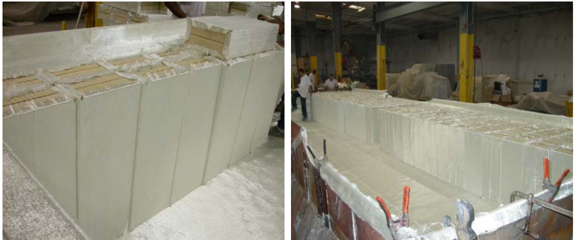
Figure 5. Installation of FRP wrapped foam bottles
