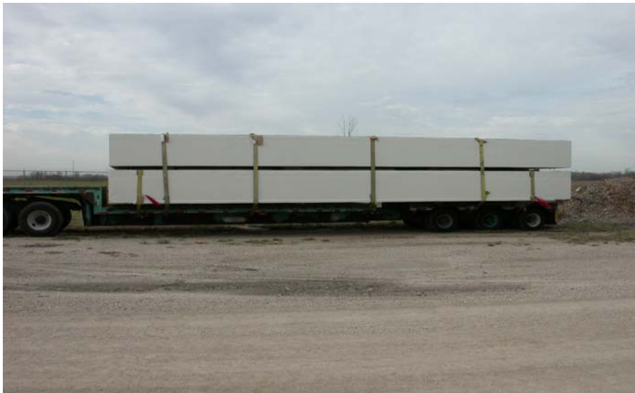
Figure 10. Delivery of Iowa DOT composite bridge.
