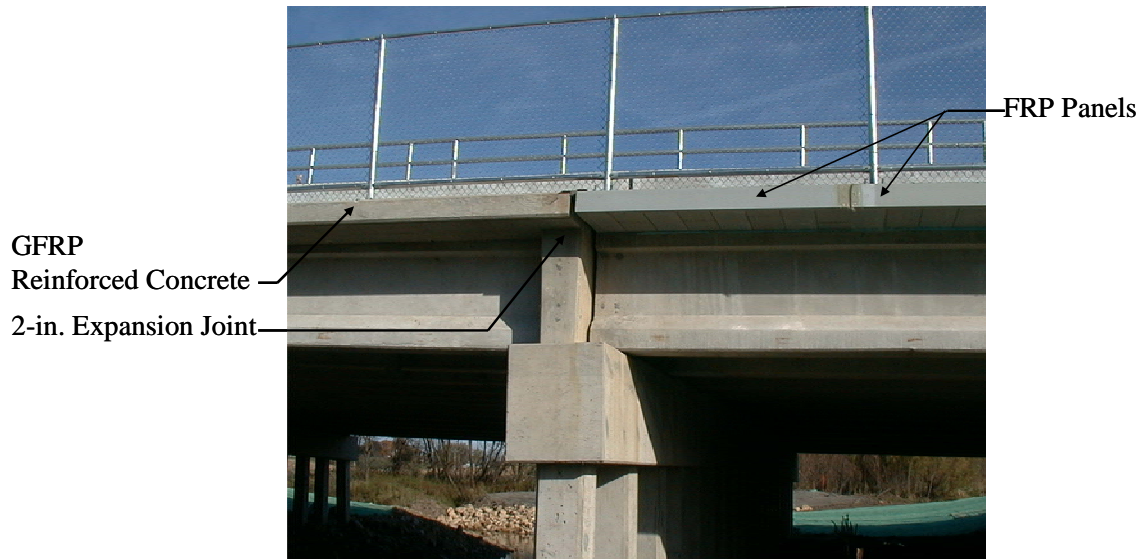
Figure 7. Expansion Joint Detail
