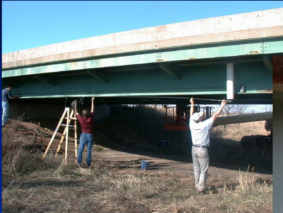
Placement of CFRP Rod
